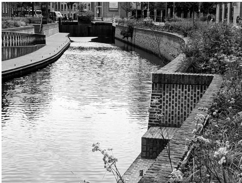
Figure 1: View of the river Mark after refurbishment during the Green-Quays project, Breda. Photo: Veerle Hemerik, 2024.
