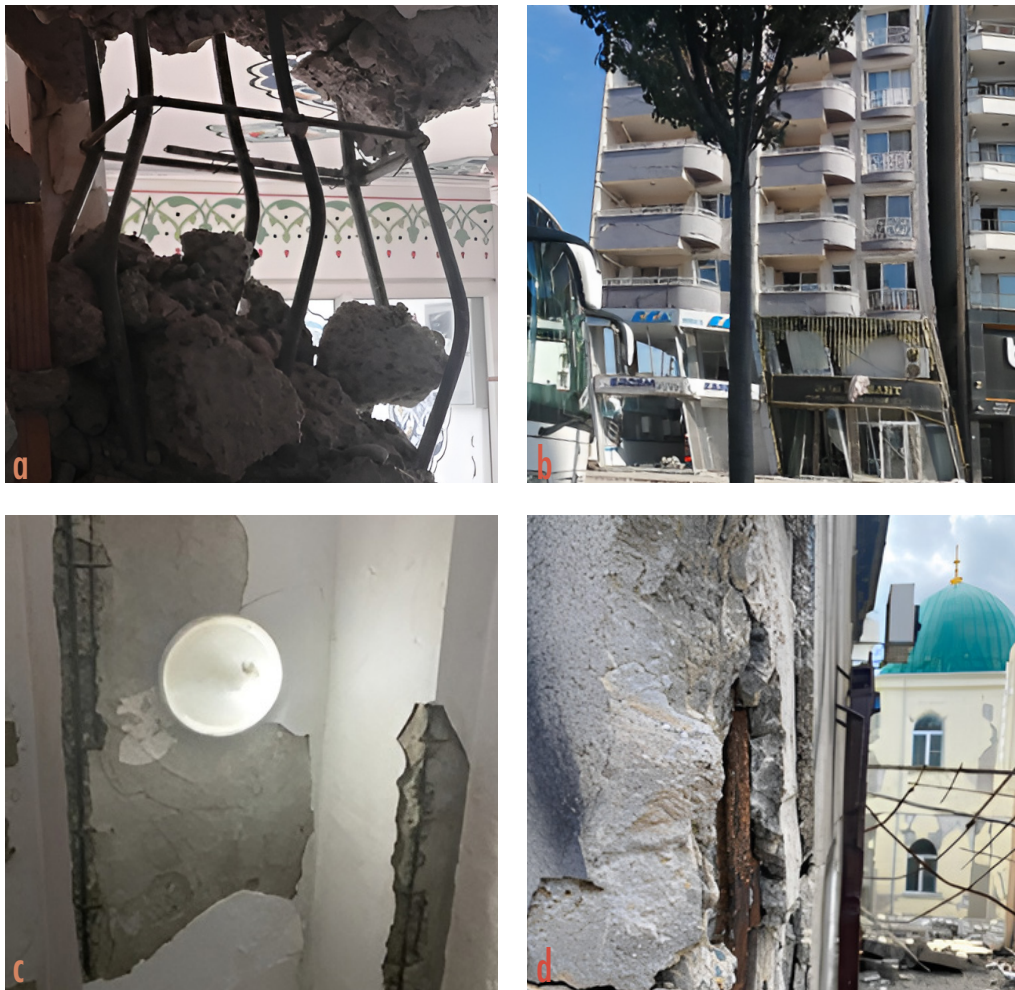
Figure 1. Some representative observed damages: (a) insufficient stirrup spacing/detailing, poor quality of concrete, lack of confinement for plastic hinge region, (b) soft & weak story formations resulting in significant lateral drift, (c) heavy corrosion in a stadium column, (d) usage of plain reinforcing bars (Images by author).
