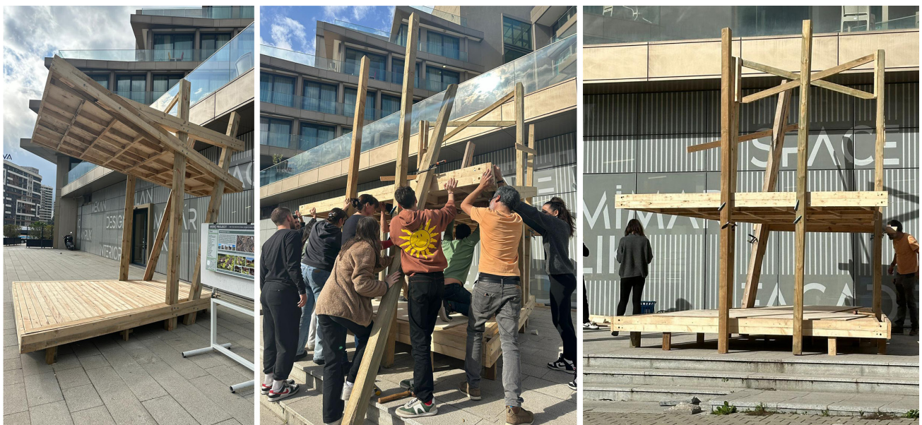
Figure 13. Process of disassembling the prototype.
