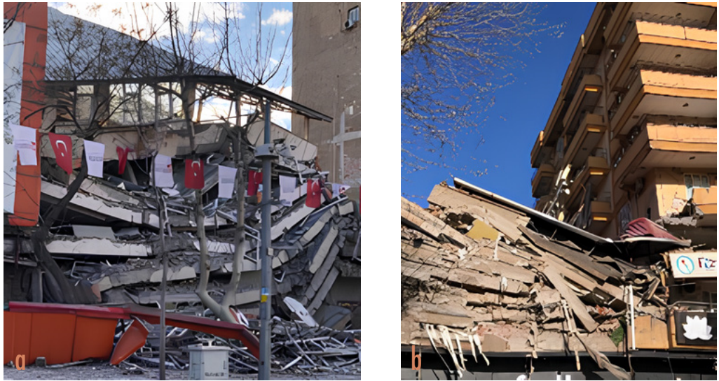
Figure 3. Examples of (a), (b) pancake collapse (Images by author).
