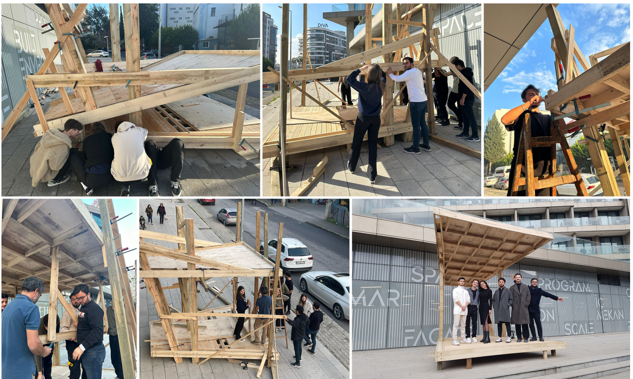
Figure 12. Raise and assembly of the roof structure.
