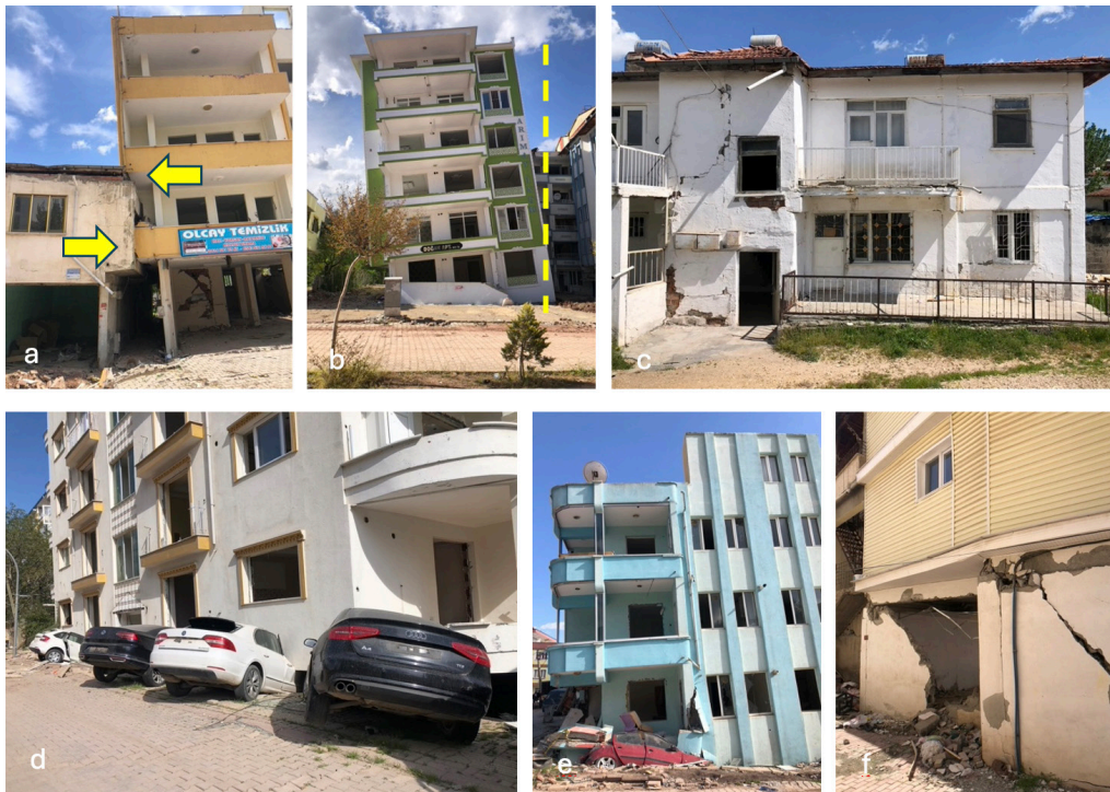
Figure 3. Soil based building damage at Golbasi a)Pounding b)Soil failure causing tilting c)Prefabricated low-rise house with repairable damage d)Soil failure (loss of ground story) e)Soil failure (loss of ground story) f)Typical infill wall-frame damage.
