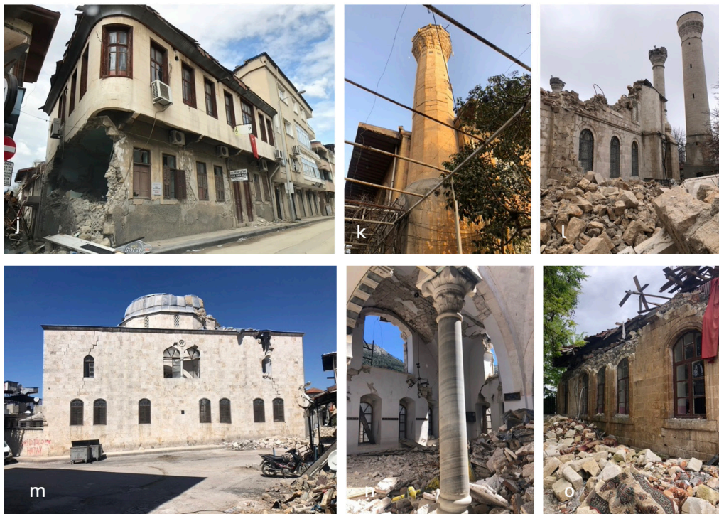
Figure 4. Continued j)Ground story wall collapse k)Minaret collapse and loss of integrity of body stones l)Mosque total collapse m)Excessive damage to newly restored mosque n)Interior view of mosque (collapse of dome and arches) o)Collapse of upper story and roof of school.
