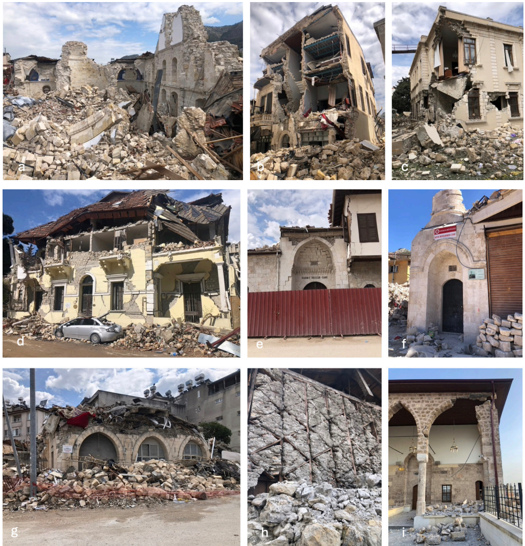
Figure 4. Masonry building damage and collapses a) Collapse of church b) Partial collapse of hotel c) Governor's building d) Severe damage and collapsed parts of masonry building e) Collapse and damage of mosque f) Minaret collapse g) Church collapse h) Limited damage to traditional building with masonry and wooden components i) Excessive damage to newly restored mosque (tie-bar fracture, arch collapse from front view-roof and other interior parts collapsed).
