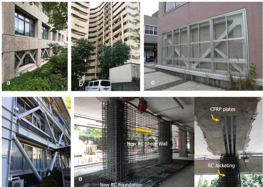
Figure 7. Real-life retrofit examples a) Adding steel bracing (Municipality Building, Japan) b) Adding seismic damper on building façade (Japan) c) Adding steel bracing (Tsukuba University, Japan) d) Adding steel dampers on building façade (TIT, Japan) e) Adding RC shear wall, new foundation, RC jacketing and using CFRP plates as reinforcement (School building, Istanbul).
