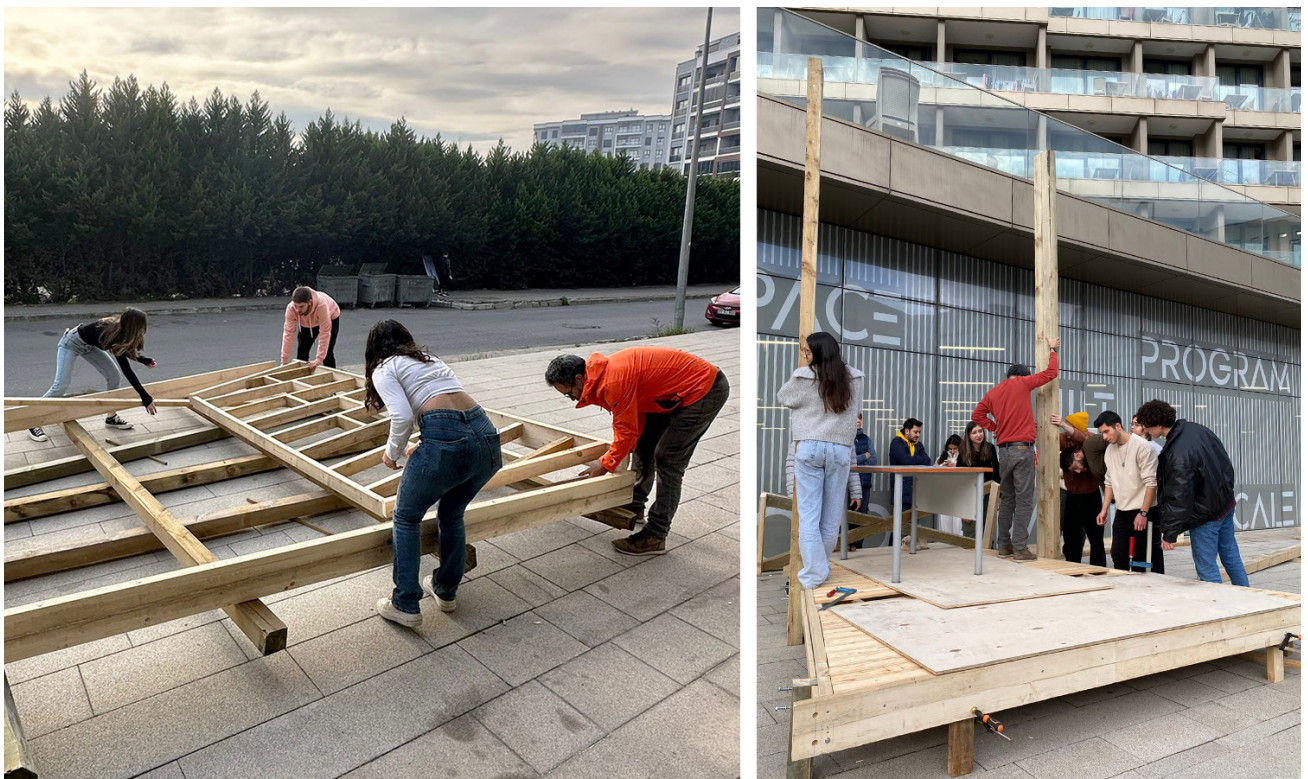
Figure 11. Assembly of floor structure and columns.
