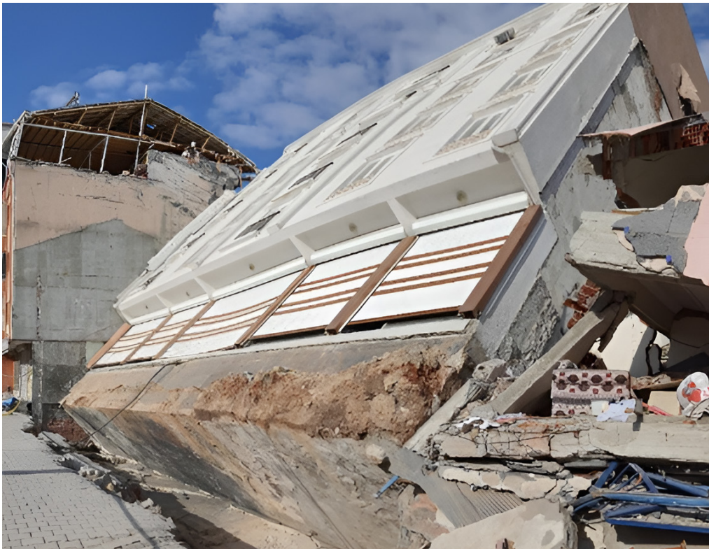
Figure 2. Example of soil liquefaction (Images by author).
