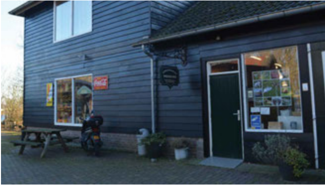
Entrance | needs improvement
