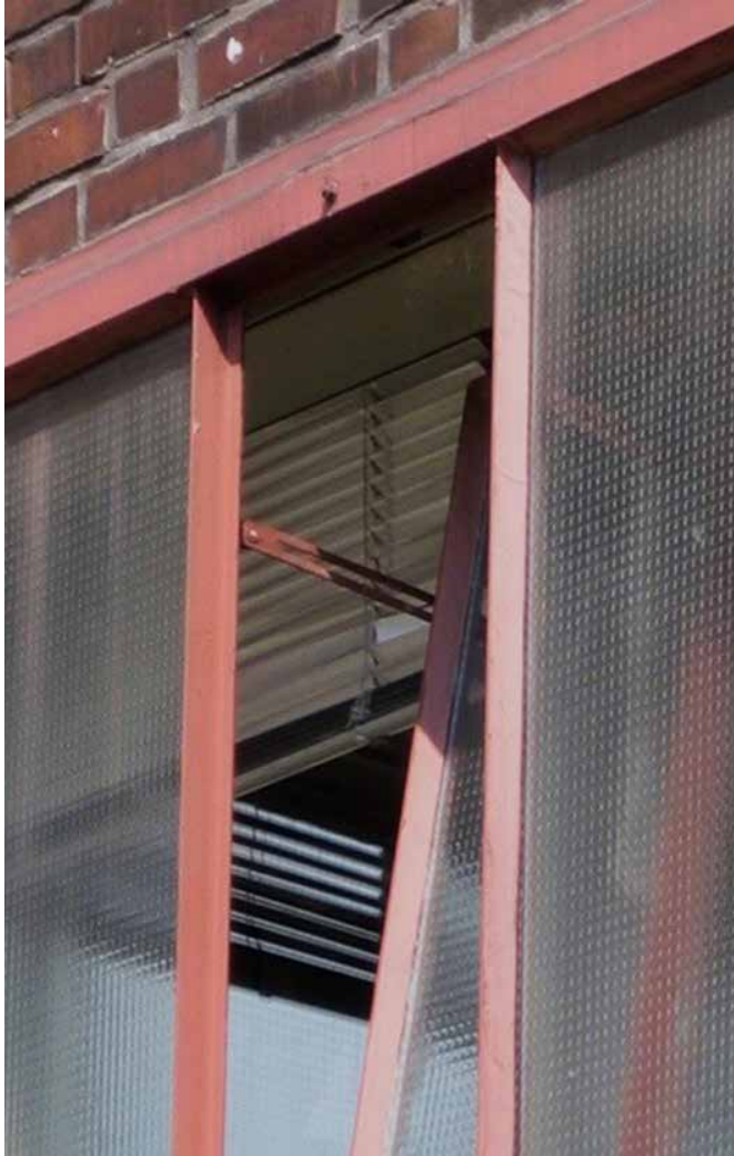
FIG. 5.21 Metal framed windows were used in industrial architecture since 18 th century, and became standard in 20 th century with mostly patterned or wired glass, Zollverein Coalmine, 1932 / Photo: U. Pottgiesser
