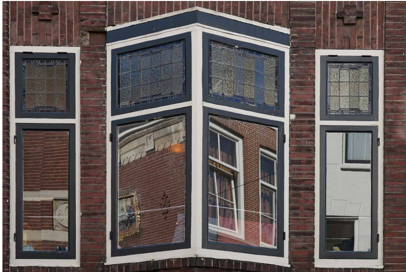
FIG. 5.1 Historic glazing / Photo: M. Olmeda
