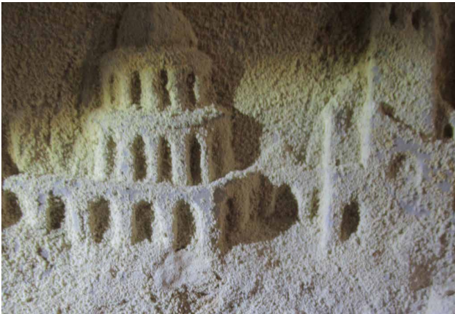
FIG. 4.5 Powdering of the stone: a consolidation treatment may be effective in this case / Photo: B. Lubelli
