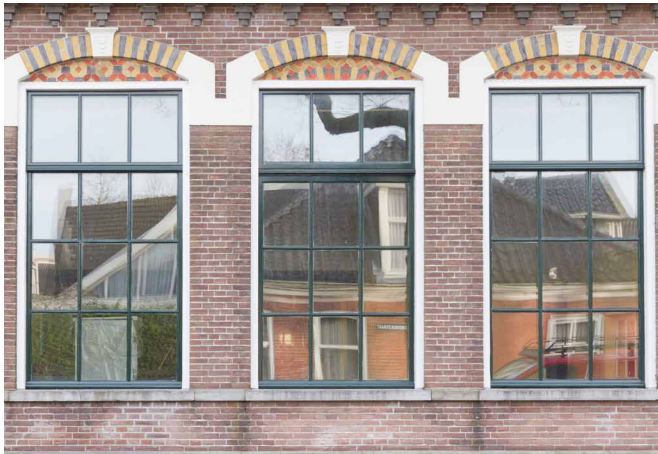
FIG. 5.17 Wooden window with muntins (glazing bars) connecting small glass panes / Photo: RCE
