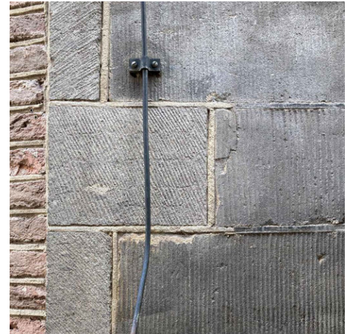
FIG. 2.7 Peperino Duro (left) used to replace Bentheim sandstone (right) in the Nieuwe Kerk in Amsterdam / Photo: W.J. Quist
