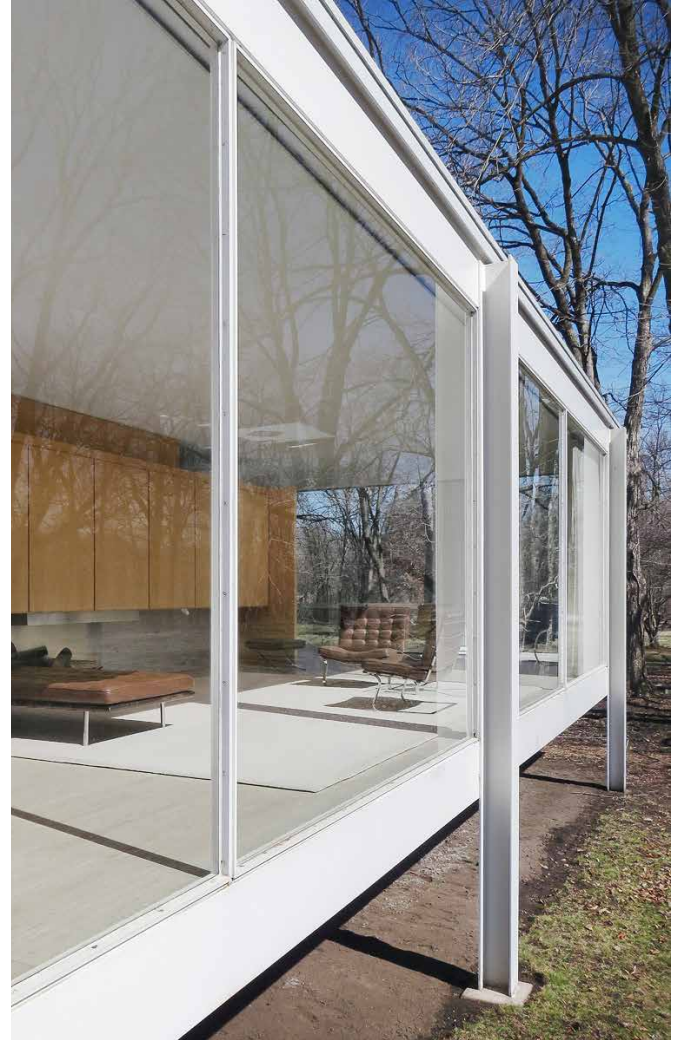
FIG. 5.22 Large metal framed windows were introduced to residential architecture in early 20 th century, and became famous with buildings like the Farnsworth House, 1951 / Photo: A. Ayón
