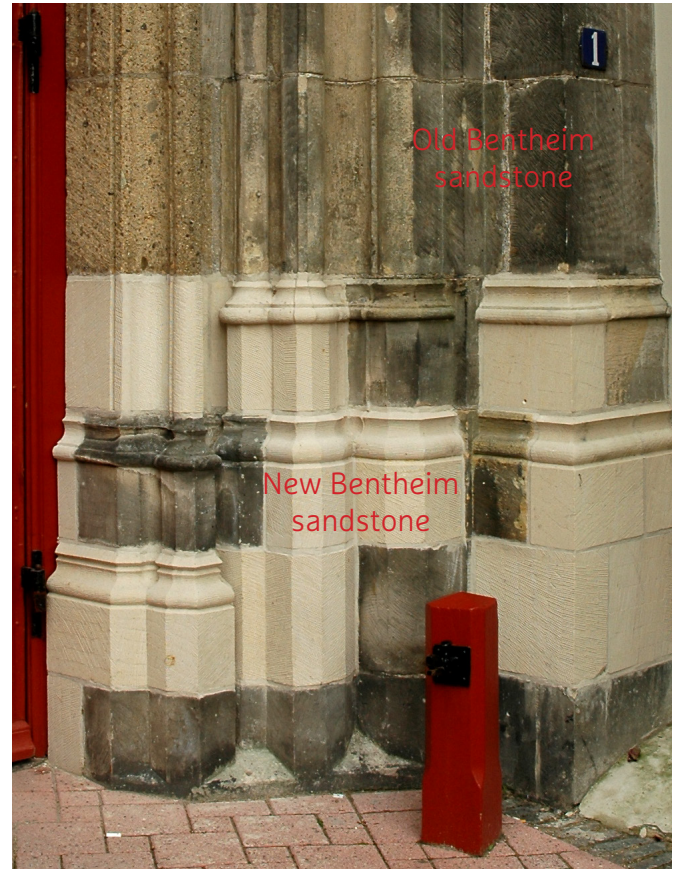
FIG. 2.11 Bentheim sandstone at the south portal of the Sint-Joriskerk Amersfoort / Photo: W.J. Quist
