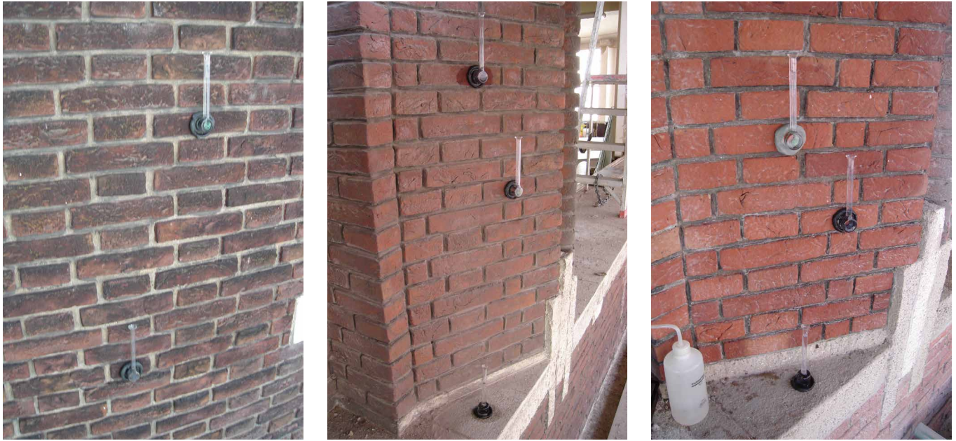
FIG. 4.27 Execution of the Karsten Tube tests on the masonry not cleaned (left), cleaned (middle) and cleaned and treated with a water repellent (right) / Photos: B. Lubelli
