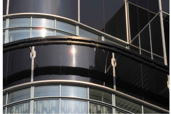
FIG. 5.10 Vitrolite spandrels at former Daily Express building by Ellis and Clark, 1932, London / Photo: https://en.wikipedia.org/wiki/Daily_Express_Building,_London#/media/File:Express_Building.jpg , accessed Aug. 2021
