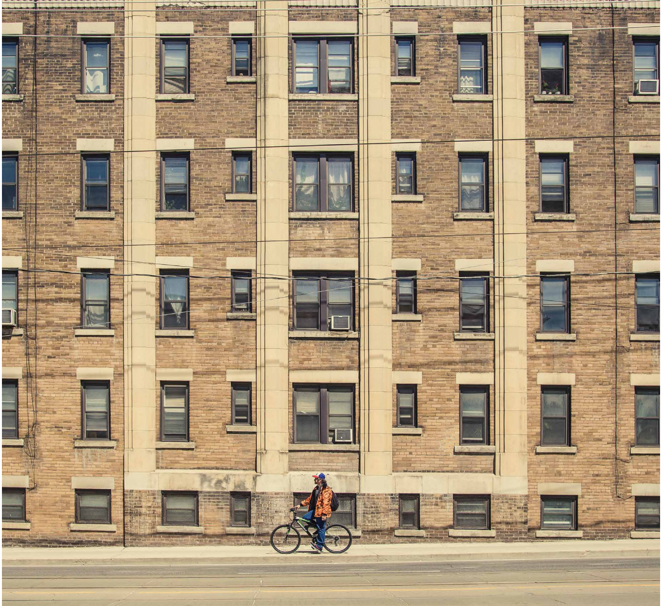
FIG. 5.19 Wooden frames were the most common material for residential buildings until mid 20 th century. From early 20 th century onwards larger glass panes were used in residential architecture / Photo: pxhere.com
