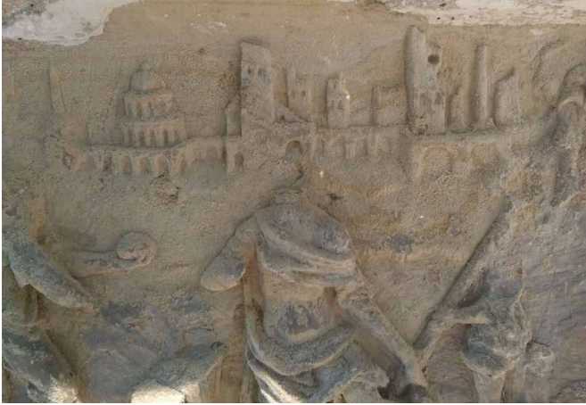
FIG. 4.4 Powdering of the stone: a consolidation treatment may be effective in this case / Photo: B. Lubelli
