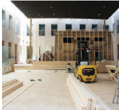
2. Temple is covered before asbestos removal
