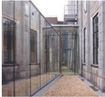
2. Henket extension (l) and old building (r)
