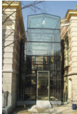
2. The glass joint forms a connection between old and new
