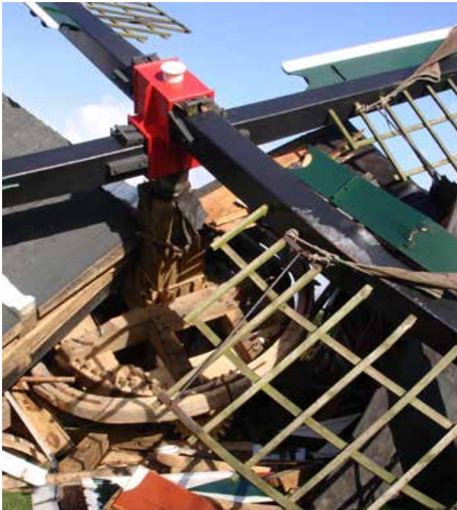
FIG. 2.3 Windmill 'Zeldenrust', Geffen. Demolished by the storm Kyrill in 2007 and rebuilt afterwards.
