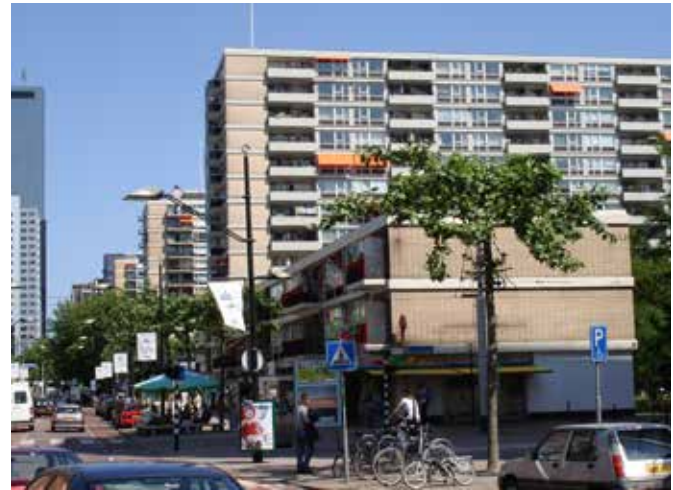
FIG. 1.7 Monument of everyday life: shops and apartments of the Lijnbaan (listed in 2012).
