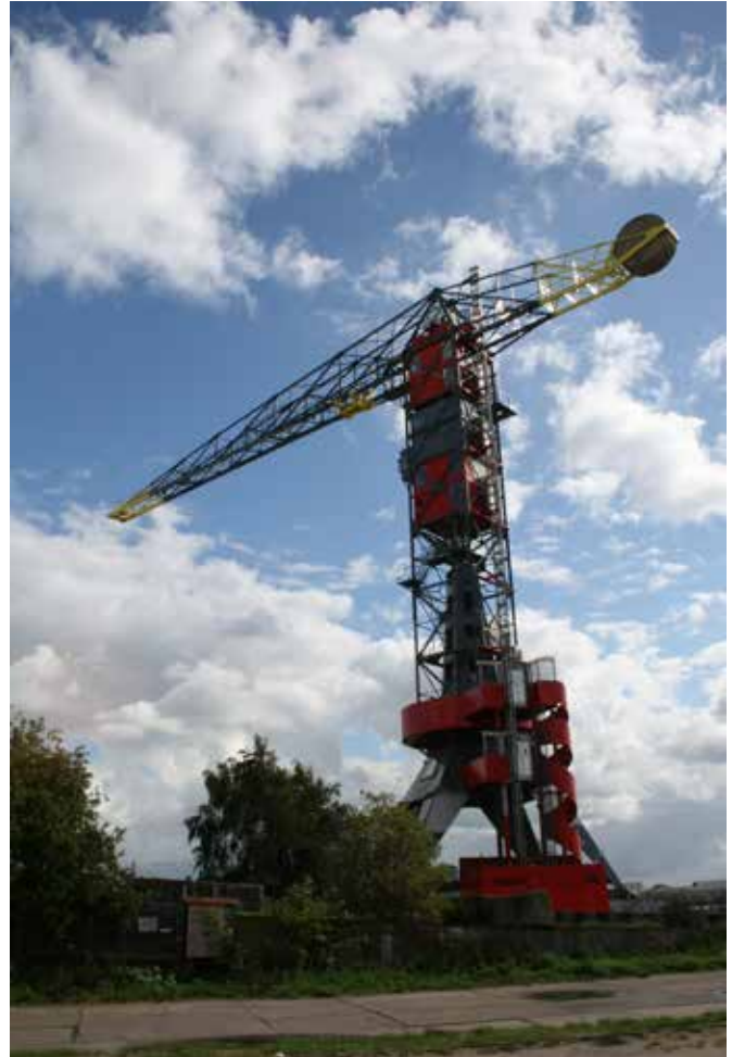
FIG. 3.87 Faralda Crane Hotel, NDSM-shipyard, Amsterdam, 2014.
