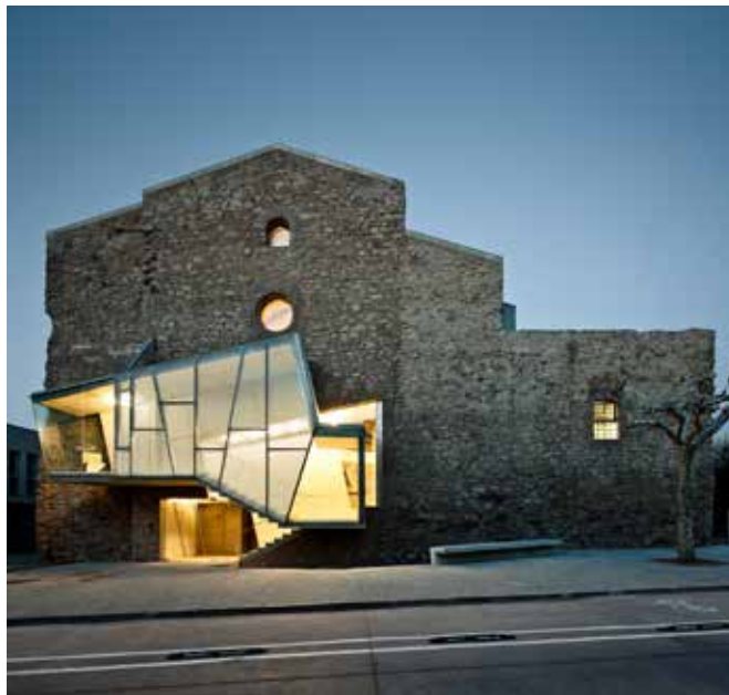
FIG. 2.22 The Convent of San Fransesc in Santpedor has been transformed into an auditorium by David Closes / Jordi Suroca
