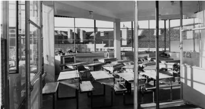
FIG. 5.30 Duiker understood that the only way to heat the (largely) open-air class rooms was to rely on radiation; he had heating pipes embedded in the reinforced concrete floors to make them act as radiation panels / W. J. van Berselen, Stadsarchief Amsterdam
