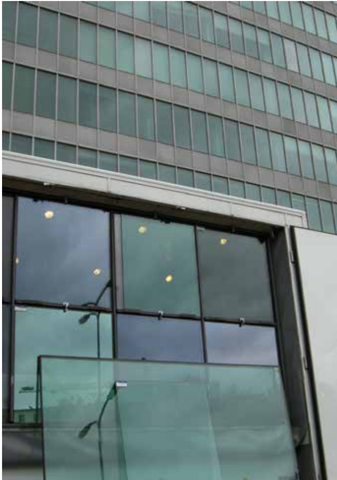
FIG. 5.35 Mock-up of various types of replacement glazing for the GAK Building; the original curtain wall in the background still features the original dark green double glazing / Wessel de Jonge Architects
