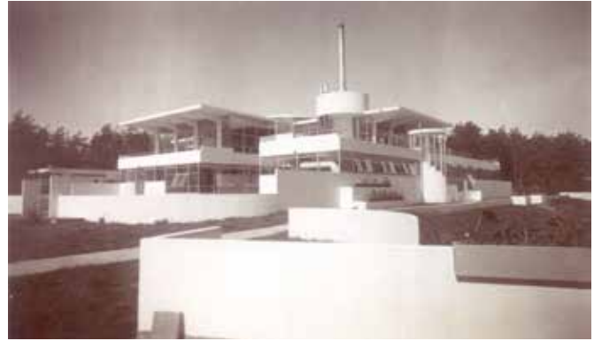
FIG. 2.7 Sanatorium 'Zonnestraal' shortly after completion in 1928. The height of the spandrel depended on the use of the space behind it. / author: unknown - International Institute for Social History
