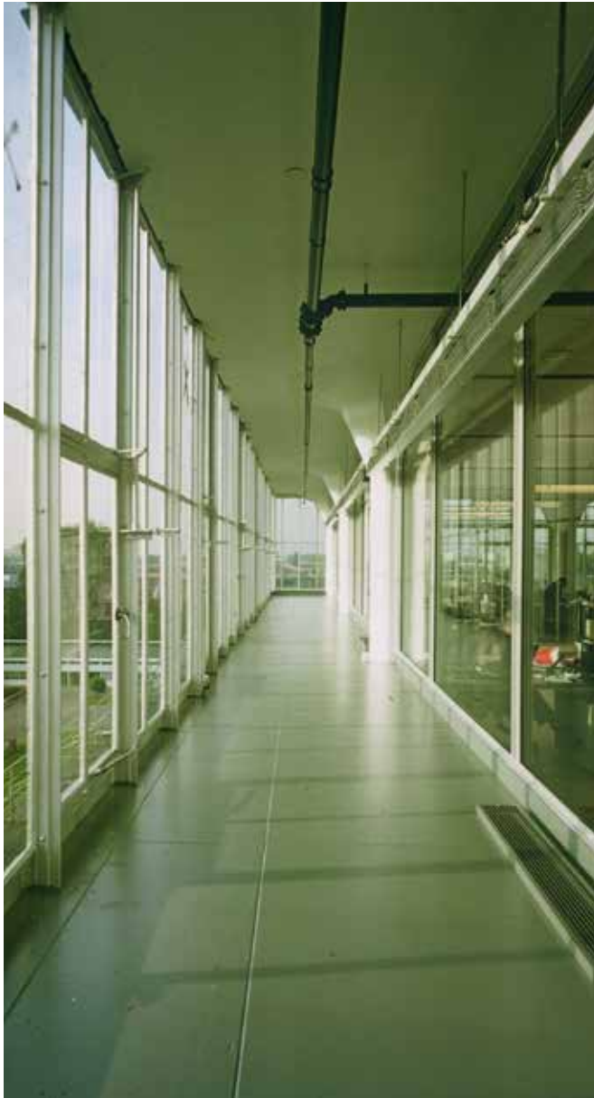
FIG. 5.27 A view inside the 'climate wall' at the western side, where solar heat gains are used during winter to pre-heat ventilation air before entering the workspaces / Fas Keuzenkamp
