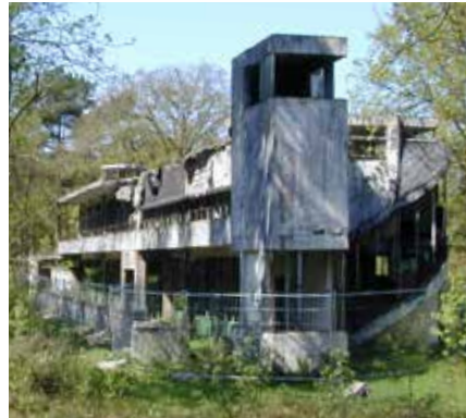
FIG. 2.9 The Dresselhuys Pavilion in 2008 after the roof had collapsed / Rudolf Wielinga,
