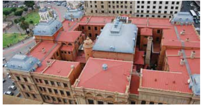
FIG. 3.21 The roof of the administrative buildings of Old Raadsaal by the Dutch-born architect Sytze Wierda located on Church Square, Pretoria / Marieke Kuipers
