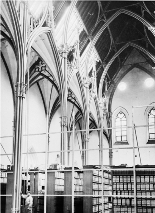
FIG. 4.6 The Great Hall (before it was reinvented as the Knight's Hall) adapted by Willem Rose through the introduction of cast iron 'Gothic' arches for the new use as the State's Archive at the Hague, about 1860 / photo: courtesy of the Cultural Heritage Agency of the Netherlands
