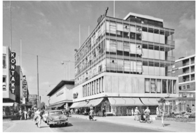
FIG. 5.15 Due to the lack of exterior sun screens, tenants of the HUF Building's office floors soon covered the windows to block out direct sunlight and added ventilators in order to minimise the excessive overheating of the interior spaces / Gemeentewerken, Gemeente Archief Rotterdam
