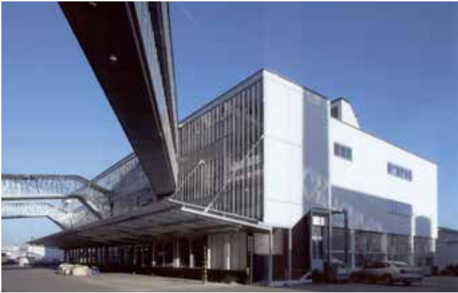
FIG. 5.6 The completion of the Dispatch Building in 1931 marked the last phase of implementation of the masterplan and is therefore part of the original state. The building was restored in 2003 / Fas Keuzenkamp
