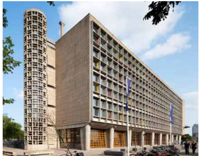
FIG. 5.22 An overview of the Technical School Patrimonium after restoration in 2013, showing the sectional doors of the former car mechanics workshop / Raoul Suermondt
