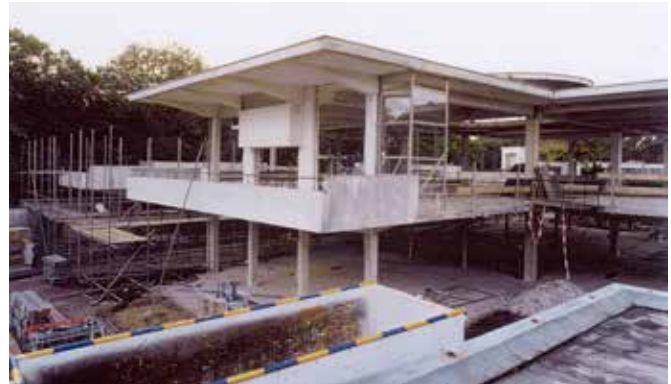
FIG. 2.16 After the removal of all later additions and alterations, this was all that was left of the original substance of the Main Building of Sanatorium 'Zonnestraal'. The upper corner shows the first test for the new glazing / Wessel de Jonge Architects
