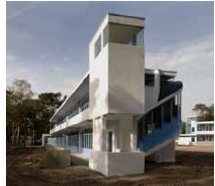
FIG. 2.10 The Dresselhuys Pavilion of 'Zonnestraal' after restoration in 2013 / Arie den Dikken
