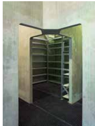
FIG. 2.20 View through the diagonally perforated silos that today accommodate an architectural archive collection / Christof Lackner
