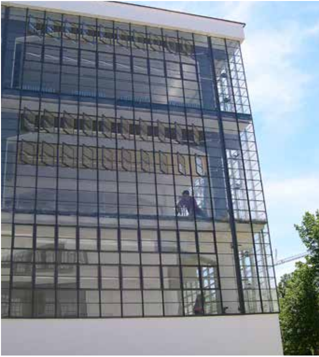
FIG. 3.17 The Bauhaus Main Building, Dessau, by Walter Gropius with its – partly reconstructed – curtain wall / Marieke Kuipers
