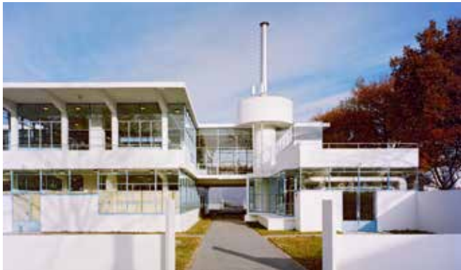
FIG. 2.15 The Main Building of Sanatorium 'Zonnestraal' after restoration in 2003 – a representation of the original idea and design intent, rather than original materials / Michel Kievits - Sybolt Voeten
