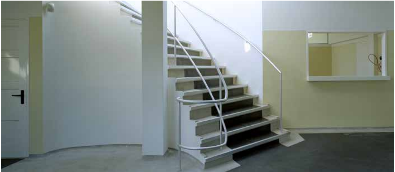
FIG. 5.10 The restored entrance lobby with remade 'expensive' linoleum and handmade cement plinths. The original linoleum was intended to reduce the noise of footsteps and the cement plinths were employed to save budget. During restoration the cement plinths had to be remade by hand at high cost / Jannes Linders
