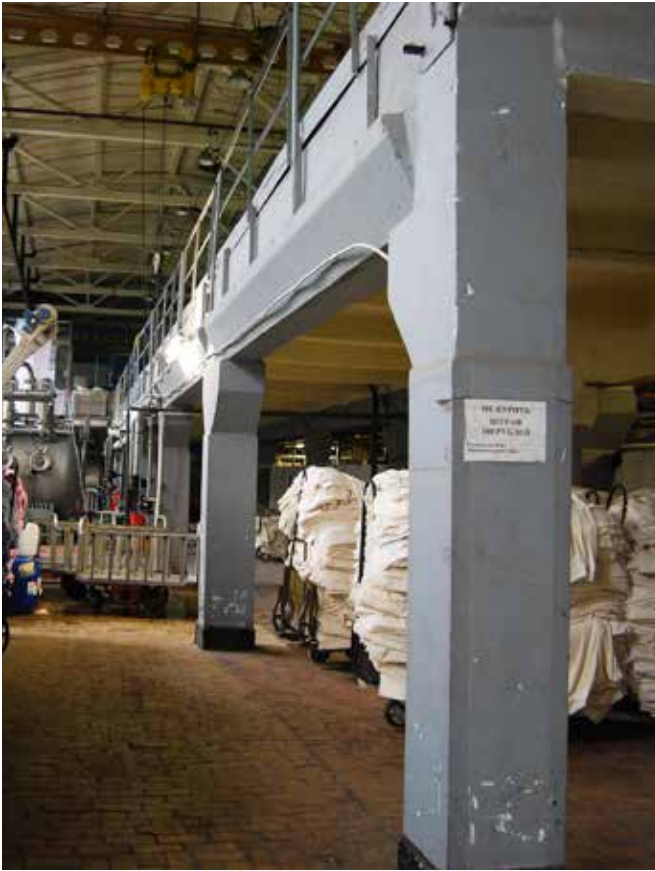
FIG. 3.27 The combined concrete frame and steel trussed structure of a former textile factory, Vishny Volochok / Marieke Kuipers
