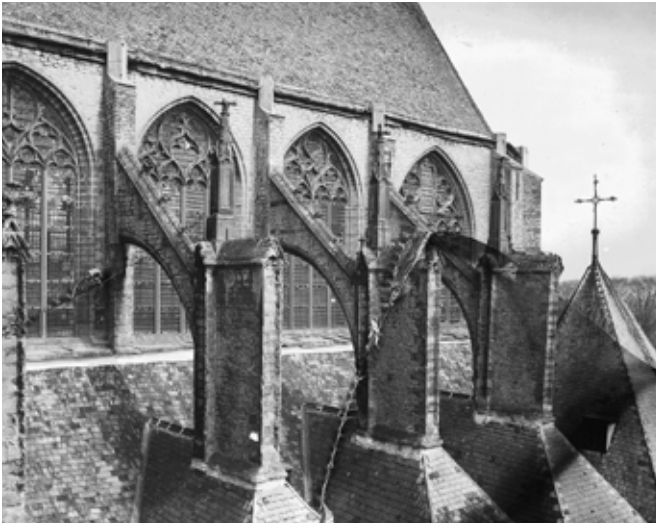
FIG. 3.30 The Gothic buttresses of the Maria Magdalena Church in Goes, photographed in 1900 / courtesy of the Cultural Heritage Agency of the Netherlands
