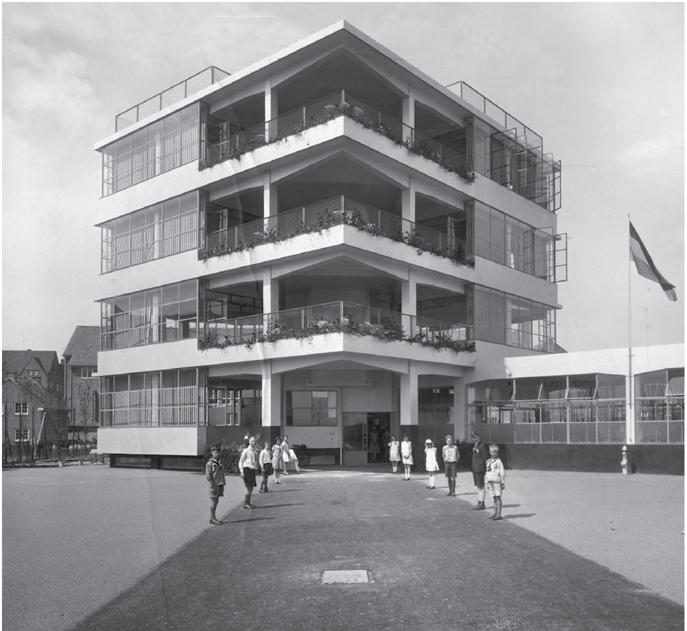
FIG. 5.29 The Open Air School in Amsterdam (Jan Duiker 1930) shortly after completion, with its the huge vertical pivot windows and terraces located on the projecting corner / Stadsarchief Amsterdam
