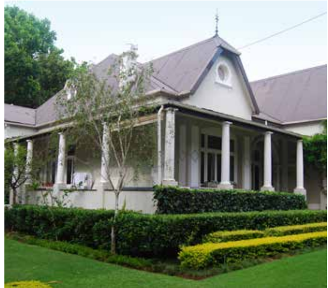
FIG. 3.10 Typical 'stoep' or veranda surrounding a house in Pretoria provides outdoor space in shade / Marieke Kuipers
