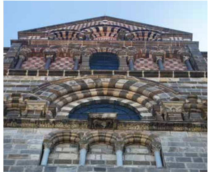
FIG. 3.26 The upper part of the façade of the Notre Dame de Puy-en-Velay, where skin and structure are inseparable / Marieke Kuipers
