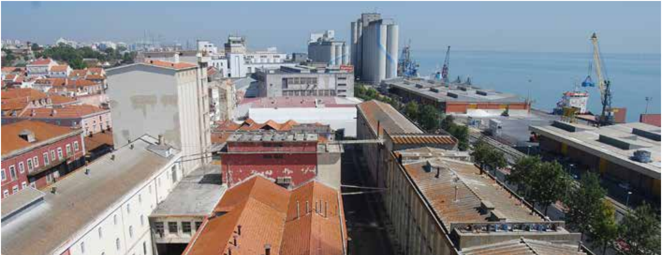
FIG. 4.16 Overview of the Manutencao Militar Complex in the parish of Beato in Lisbon, located parallel to the Tagus River as seen from the top of the complex's silo / Marieke Kuipers
