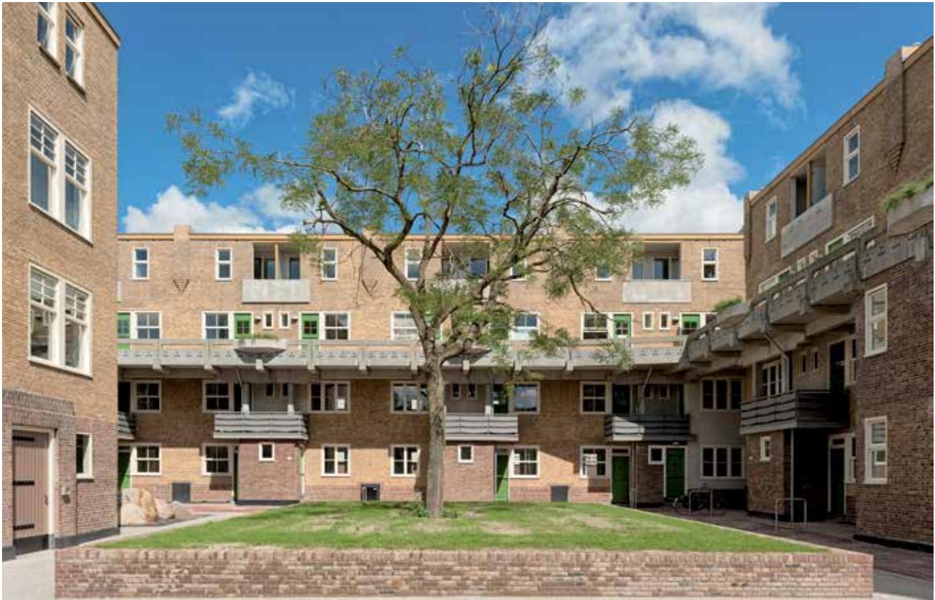
FIG. 6.16 Justus van Effen complex after restoration (Rotterdam, The Netherlands) / photo: BK Visuals Bas van Kooij
