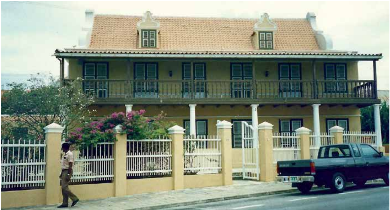
FIG. 4.1 Use of verandas for protection against the sun (mansion, Curaçao, Caribbean) / photo: R. v. Hees
