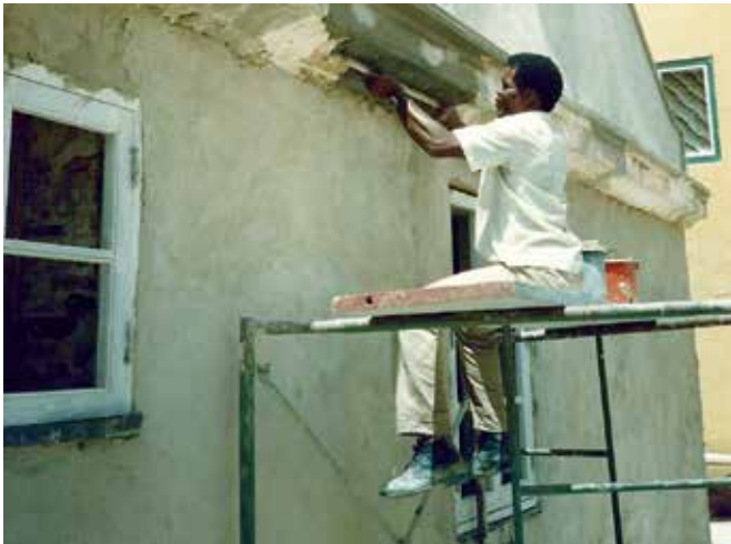
FIG. 4.2 System of aqueducts (house, Curaçao, Caribbean) / photo: R. v. Hees
