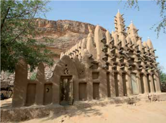
FIG. 2.5 Adobe brick construction, rendered with adobe; the wooden beams protruding from the walls are used for maintenance activities (mosque in Mali, Africa) / photo: L. Edelbroek
