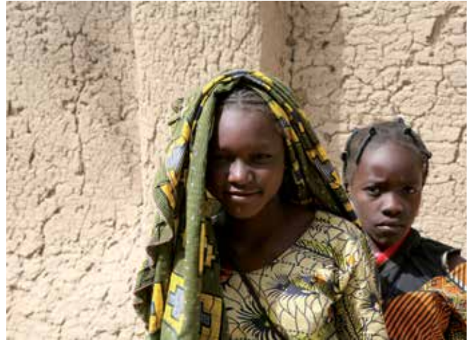
FIG. 2.6 Crack patterns, like crazing, can easily occur in the adobe rendering of external walls (Mali, Africa) / photo: L. Edelbroek
