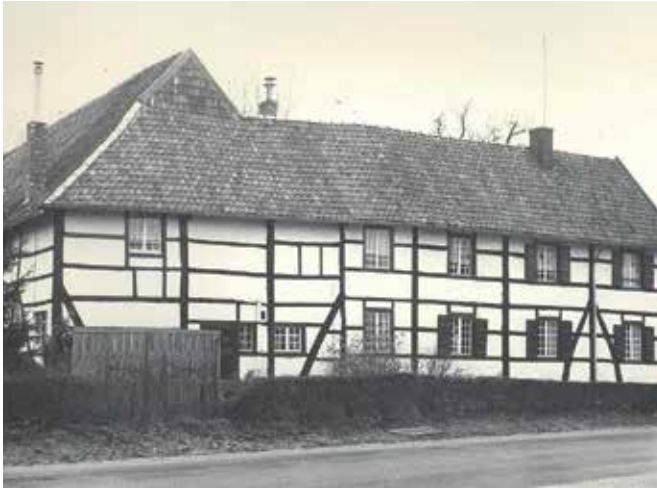
FIG. 2.20 The timber frame buildings originally had an infill of wattle and daub on a wooden lattice (house, south of Limburg, The Netherlands) / photo: R. v. Hees
