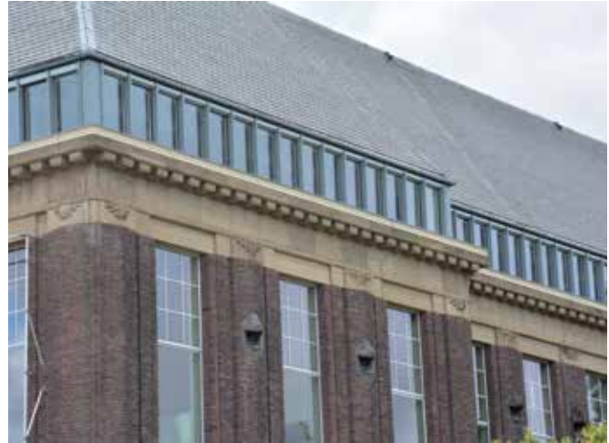
FIG. 6.31 Present situation of roof and windows; the frames are now aluminum (Faculty of Architecture, TU Delft, The Netherlands) / photo: S.Naldini
