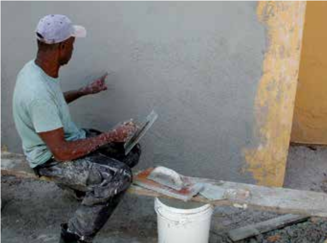
FIG. 4.13 Newly designed render compositions with assumed better salt resistant behaviour (house at Charloo, Curaçao, Caribbean) / photo: R. v. Hees
