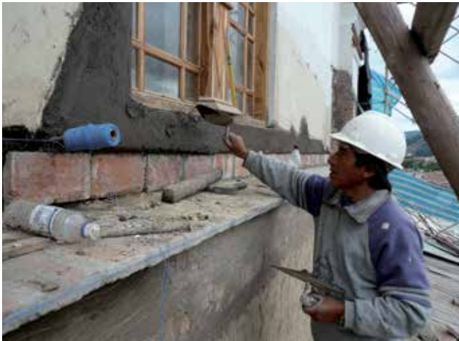
FIG. 2.10 A layer of brick masonry has been applied to better deal with the rainwater that can gather at the horizontal cornice (building in Cuenca, Ecuador) / photo: R. v. Hees
