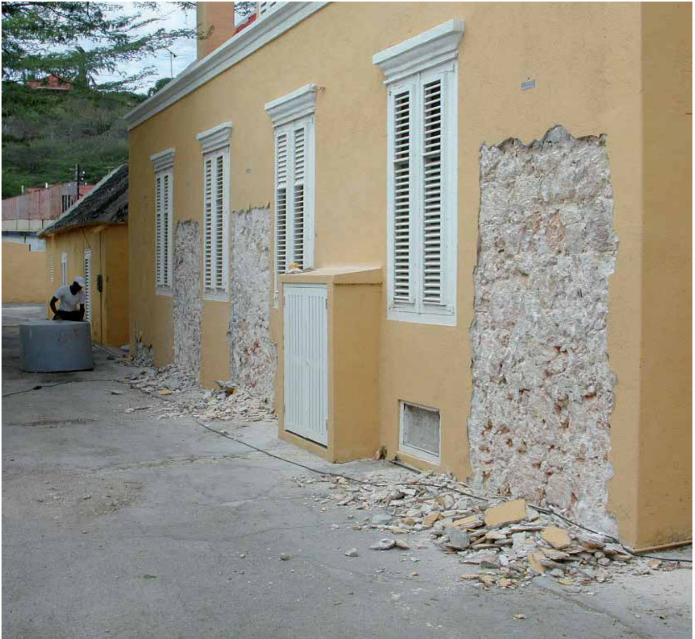
FIG. 4.12 Preparation of test panels (house at Charloo, Curaçao, Caribbean) / photo: R. v. Hees
