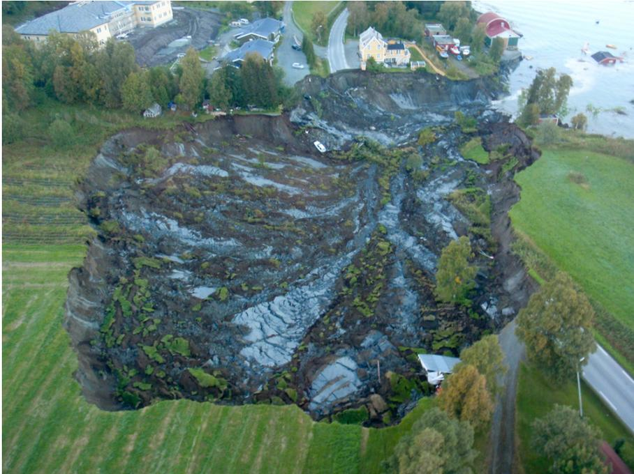
Quick clay landslide<sup>95</sup> at Lyngseidet (Norway) in 2010 (220.000 m<sup>3</sup>). The landslide was likely triggered by loading of fill along the shoreline. (See the white car in the upper part for scale)
