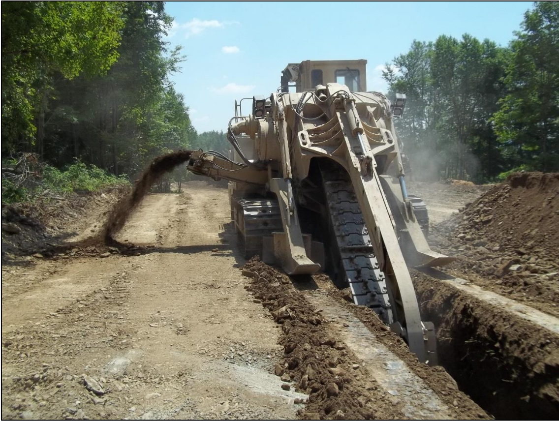
Figure Y-62: NEPA pipeline trenching (lindeco.com).
