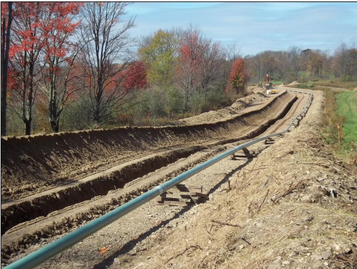
Figure Y-63: NEPA pipeline trenching (lindeco.com).
