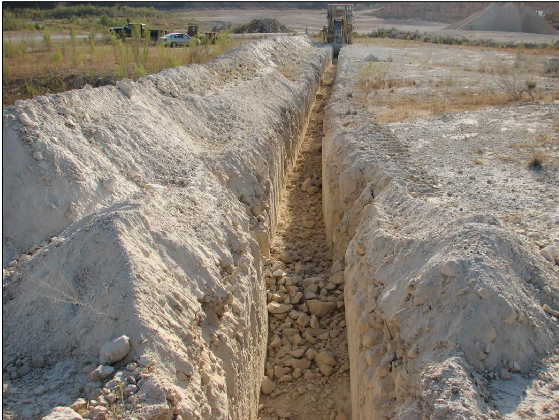
Figure Y-60: Rock trencher (Rocksaw International).
