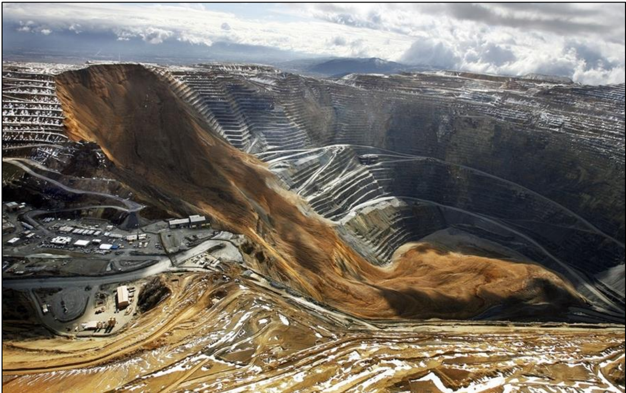
Figure 2-53: An example of active soil failure, Utah copper mine landslide (photoblog.nbcnews.com).
