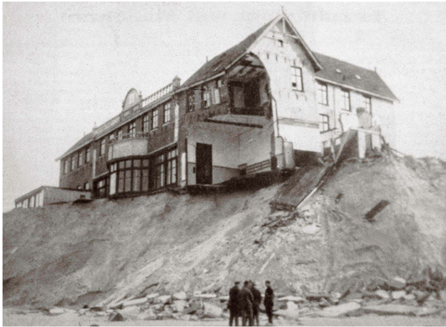
Figure 10.6: Historical photo of damage to a hotel at Schiermonnikoog due to dune erosion, circa 1923. From Rijkswaterstaat ( Credits on page 575).
