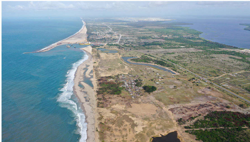
Figure 10.10: Westward-looking aerial photo of the Sandbar Breakwater, including the sand engine, Lekki, Nigeria. Image courtesy of CDR International B.V.
