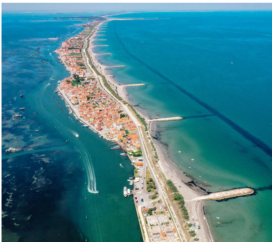
Figure 10.40: Submerged breakwater serving to perch the beach nourishment at the Pellestrina barrier island, in Venice, Italy. On the left side the Venetian Lagoon and on the right side the Adriatic Sea. Photo by Ni_Giri ( ‘Credits’ on page 575).
