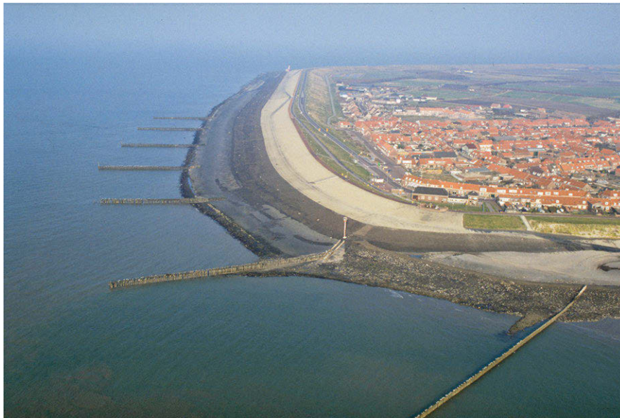
Figure 10.28: Sea dike, Westkapelle, the Netherlands, in June 1993. From Rijkswaterstaat ('Credits' on page 575).
