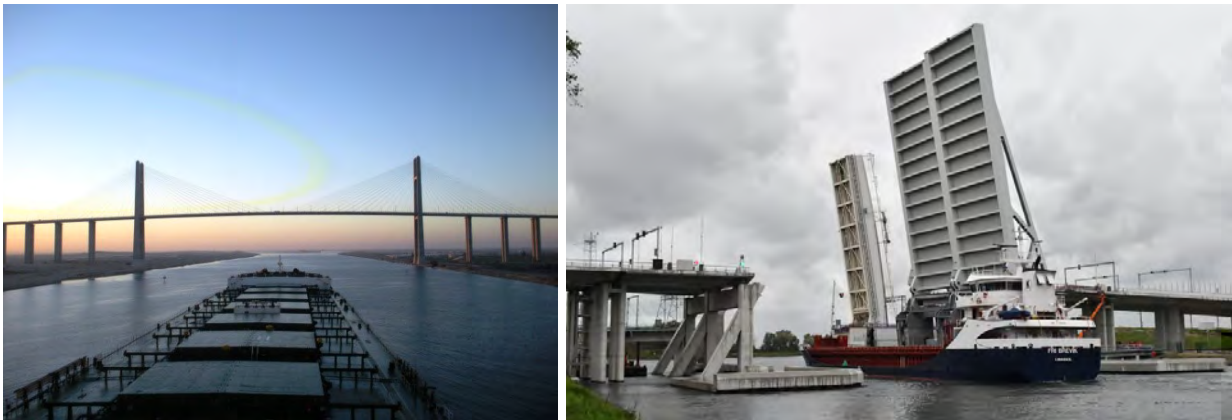
Figure 1.25: Left: Fixed bridge across the Suez Canal (by Aashay Baindur is licenced under CC BY-SA 3.0); right: Movable bascule bridge (by Tvx1 is licenced under CC BY-SA 4.0).
