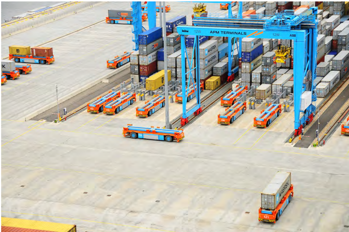
Figure 4.42: ARMG and truck transfer docks, AMPT Maasvlakte 2 (APM Terminals Maasvlakte II, Rotterdam by APM Terminals is licenced under CC BY-NC-SA 4.0).
