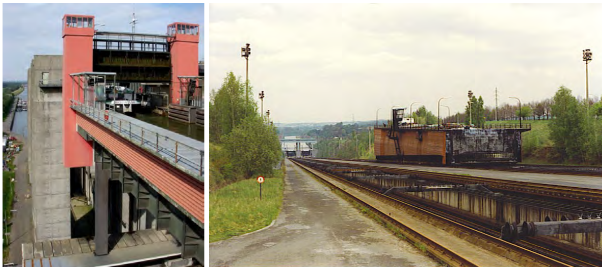
Figure 1.24: Left: Ship lift at Scharnebeck, Germany (by Holger Ellgaard is licenced under CC BY-SA 3.0); right: Inclined slope of Ronquies, Belgium (by Jean-Pol Grandmont is licenced under CC BY-SA 3.0).
