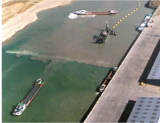
Figure 2.20: Dredging-induced turbidity containment with a bubble screen ( Turbidity & Dredging by Royal Van Oord is licenced under CC BY-NC-SA 4.0).
