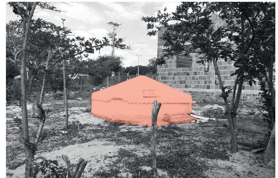
Fig. 3 Rainwater harvesting in Jaguaribara. The cistern is semi-buried to keep the water at a mild temperature until it can be manually extracted and purified for consumption. Adapted from Veras Morais (2020).
