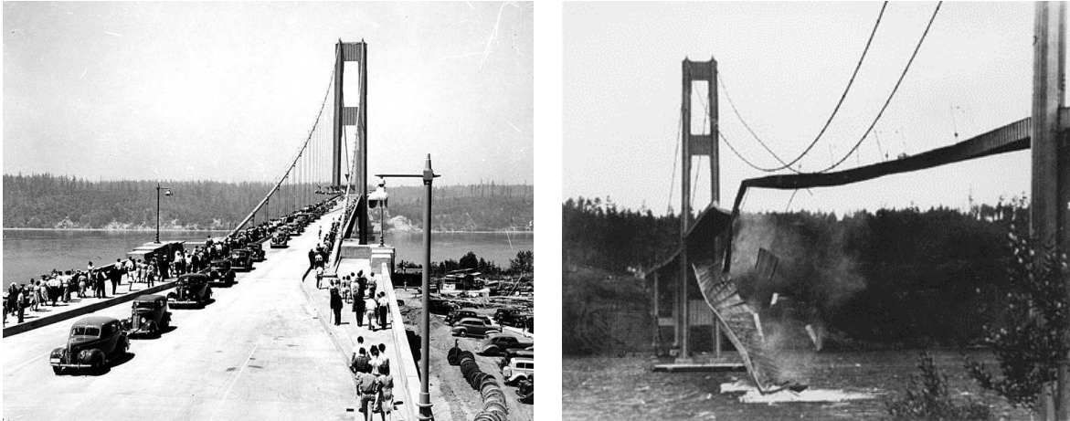
Figure 1.7: The Tacoma Narrows bridge, a suspension bridge in the US state of Washington that spanned Puget Sound, opened to traffic on July 1st, 1940, at left, and dramatically collapsed into Puget Sound on November 7th of the same year, at right, because of variable wind loads acting on the bridge deck. The Tacoma Narrows bridge is a classical and popular example of resonance in engineering, though the actual cause of the collapse was more intricate. Images taken from Wikimedia Commons and Wikimedia Commons [1], public domain.
