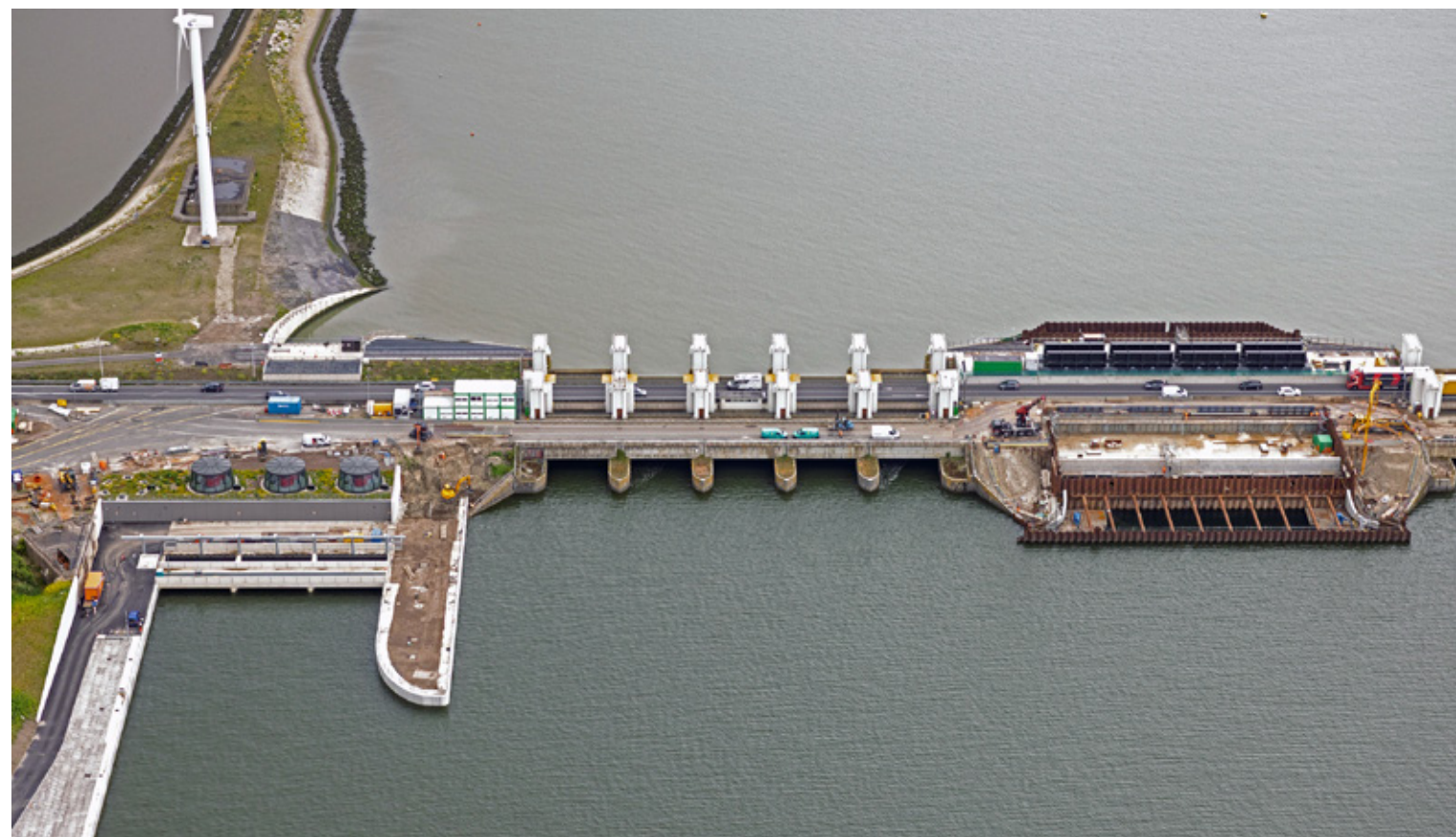
Figure 6. Left: newly developed Levvel bloc for reinforcement of the dike at the Wadden Sea side. [© Jan Wessels] / Right: application of Levvel blocs for the Fish Migration River. [© Rijkswaterstaat, Jan Wessels] / Figure 7. New pumps (left) at Den Oever sluice complex next to the existing sluice gates (middle). Additional sluice gates are under construction (right). This configuration is doubled within the entire complex. [© Levvel]
