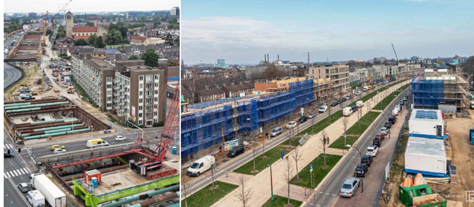
Figure 4. De Groene Loper, Maastricht: the tunnelling of the A2 contributed to the elimination of negative externalities like emissions and noise, and to positive externalities like the improvement of the living environment, higher value of existing housing and additional value of new housing development. [© Ballast Nedam / © Ballast Nedam, Aron Nijs]
