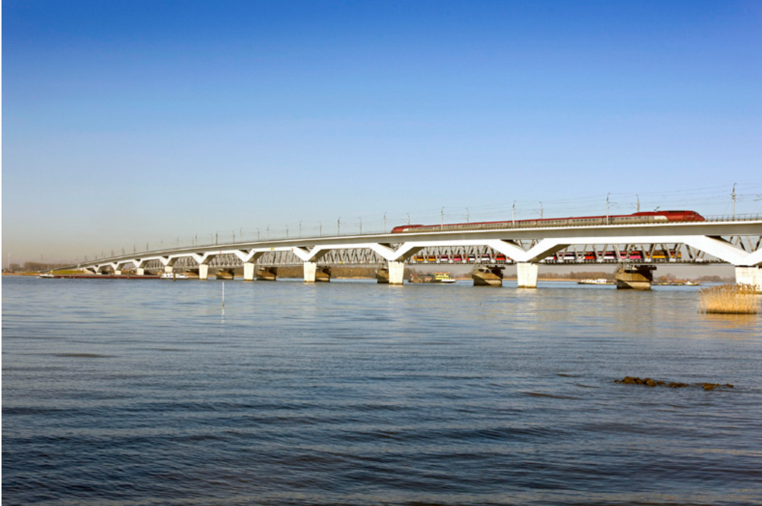
Figure 1. HSL bridge across Hollands Diep, South Holland - North Brabant: the Dutch high-speed railway project was a pioneering project for the application of systems engineering in Dutch civil infrastructure. [© Rijkswaterstaat, Joop van Houdt]
