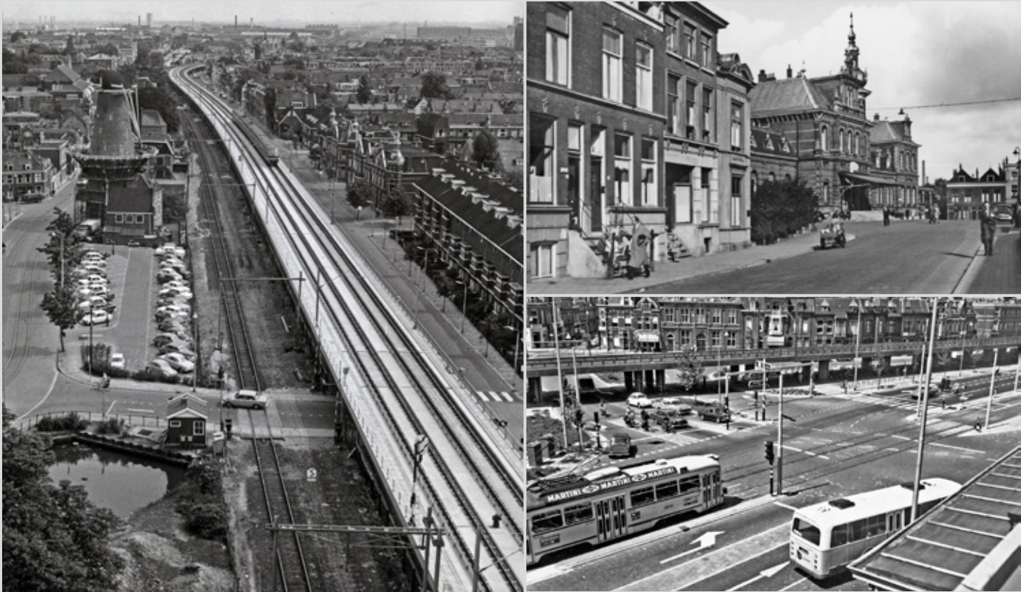
The then new railway viaduct built in 1965 near windmill De Roos, still with the original ground level tracks which were removed later. [PD Het Utrechts Archief, L. Hessels] / Now demolished townhouses at Van Leeuwenhoeksingel and the old station in 1956. [PD Stadsarchief Delft, Jospé Arnhem] / View of the railway viaduct from Westvest in the direction of Bolwerk, Spoorsingel and Phoenixstraat in 1967. [PD Stadsarchief Delft, Municipal police]
