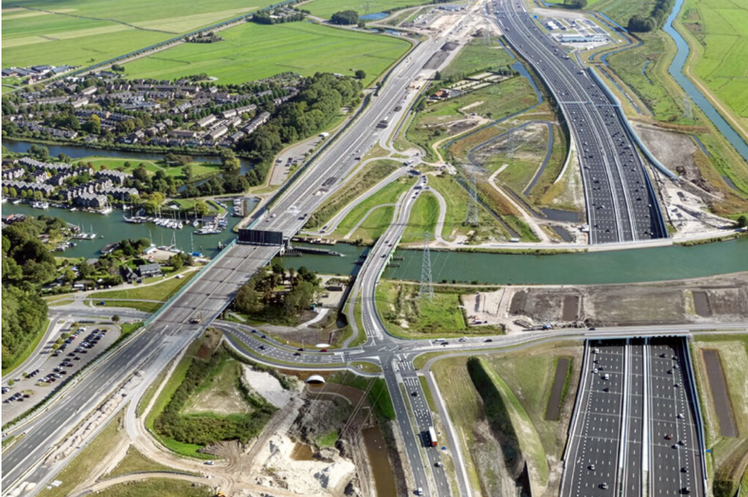
A1, Naarden, North Holland: re-routing and widening of the motorway, initially with a bridge over the Vecht River, with the road now passing under an aqueduct. [© Rijkswaterstaat] / Table 2 (below): elevation options for infrastructure. [© Jan Nederveen, Lindy Molenkamp, Enne de Boer]
