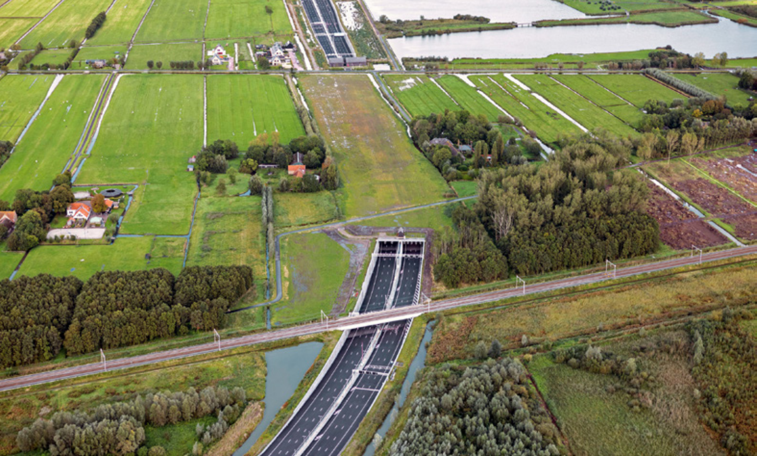
Blankenburgverbinding (A24): the Holland tunnel under the Zuidbuurt area, the viaduct of the Hoekse Lijn, and the sunken road along Krabbeplass towards the A20 on the north bank of the Nieuwe Waterweg (top). Connection of the A15 with the A24 and the Maasdelta tunnel between Rozenburg and the port on the south bank (bottom). [© Rijkswaterstaat, Topview Luchtfotografie]
