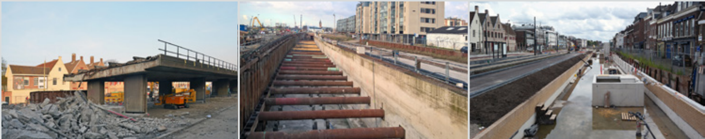
Demolition of railway viaduct. [CC Tukka] / Construction of the railway tunnel called William of Orange tunnel, referring to the historic bond of the royal family with Delft. [CC Bennie91] / Reconstruction of the former city canal and construction of parking entrances on the roof of the underground parking located on the site of the demolished viaduct. [CC Steven Lek]
