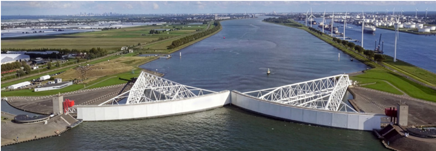
Maeslantkering, Hoek van Holland, South Holland: storm surge barrier with movable arms of 210 metres each, with a height of 15 metres, which can withstand a flood wave of 5 metres NAP. The closing time is 2 hours. [© Rijkswaterstaat, Joop van Houdt]
