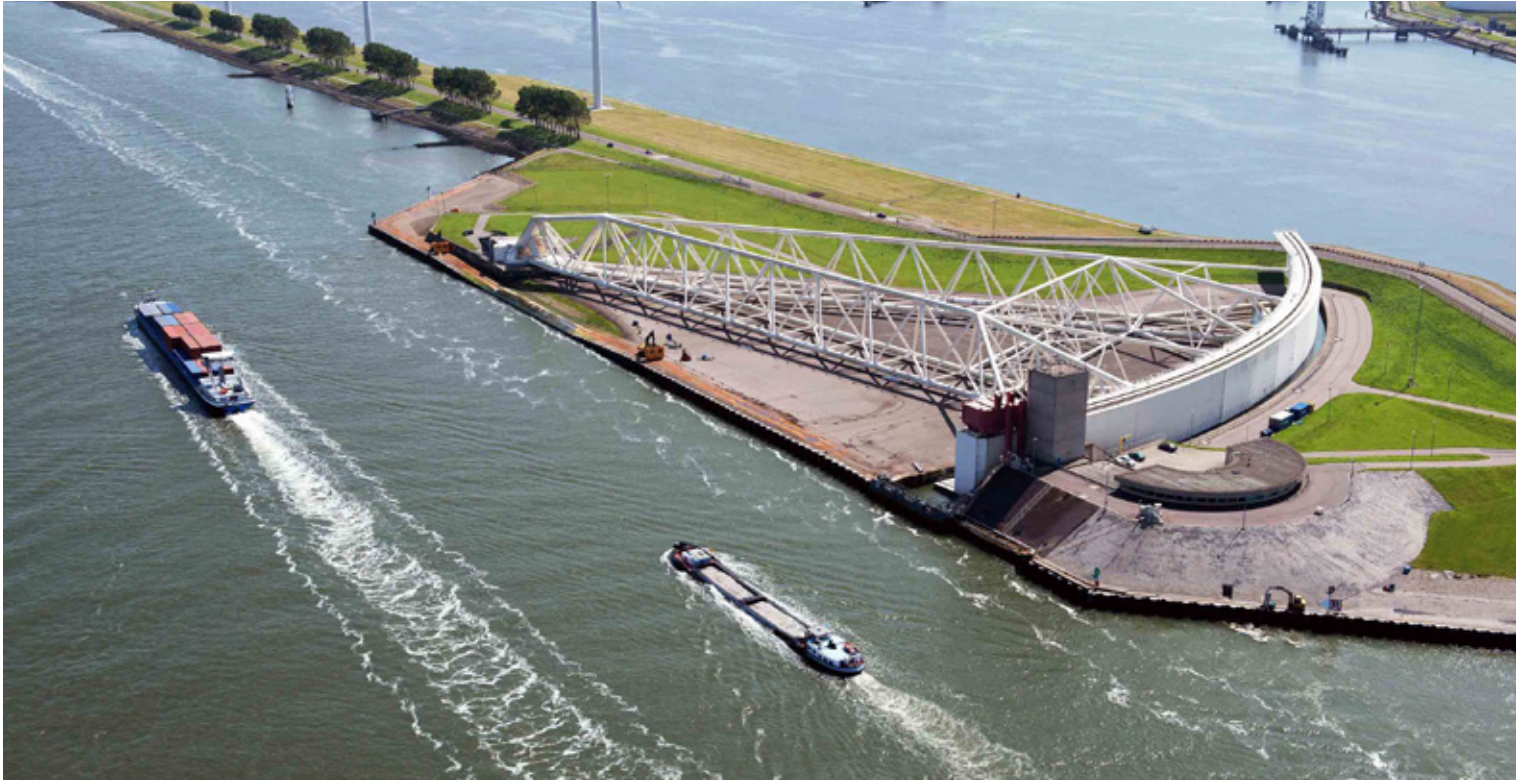
Maeslantkering, Hoek van Holland, South Holland: storm surge barrier with movable arms of 210 metres each, with a height of 15 metres, which can withstand a flood wave of 5 metres NAP. The closing time is 2 hours. [© Rijkswaterstaat, Joop van Houdt]
