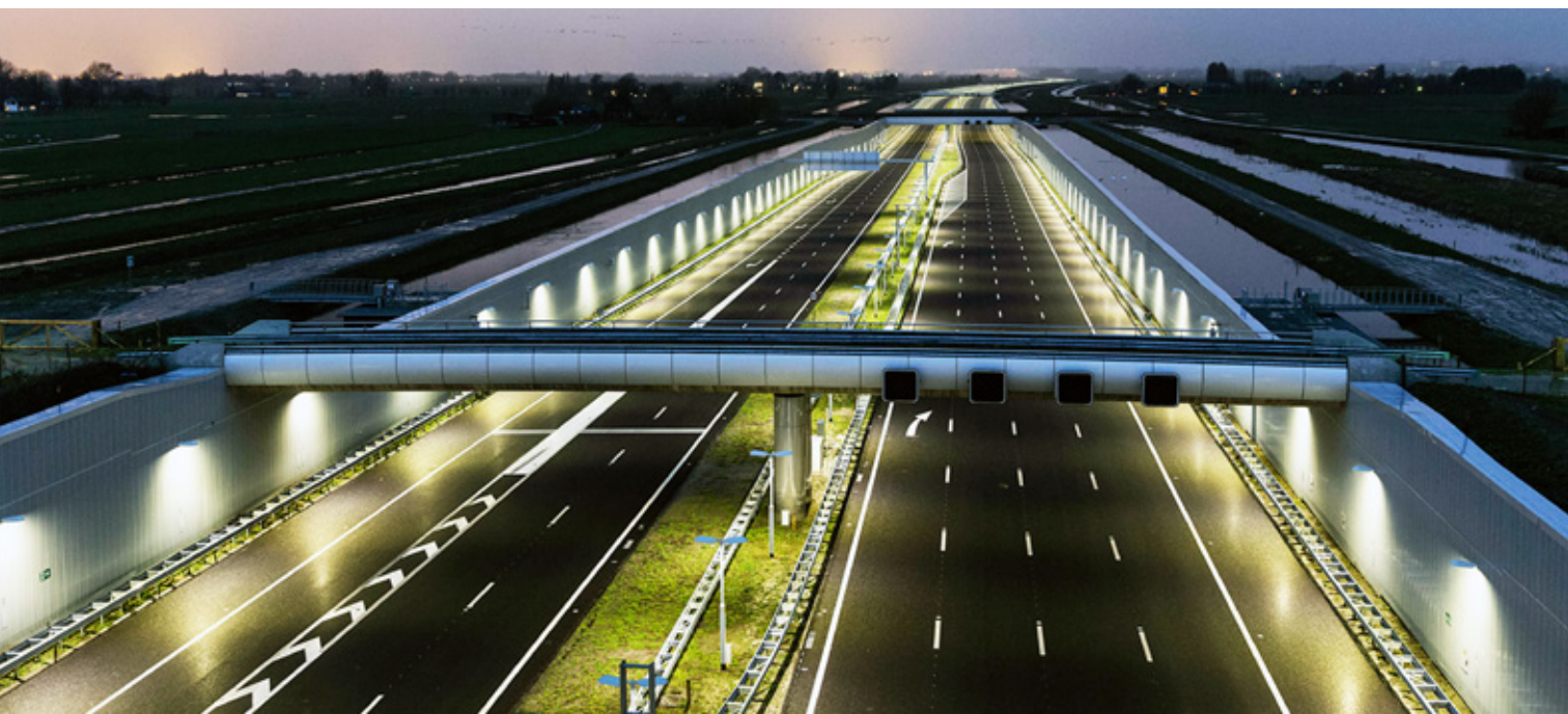
A4 Delft-Schiedam, South Holland: sunken motorway through the Midden-Delfland polder area, minimizing noise and visual disruption and maintaining waterways, with the Kethel land tunnel at Schiedam. [© Jeroen Musch (top) / © Rijkswaterstaat, Joop van Houdt (middle)] / Below: lowered lightning to reduce spill-over in the landscape. [© Heijmans, Marc Blommaert]
