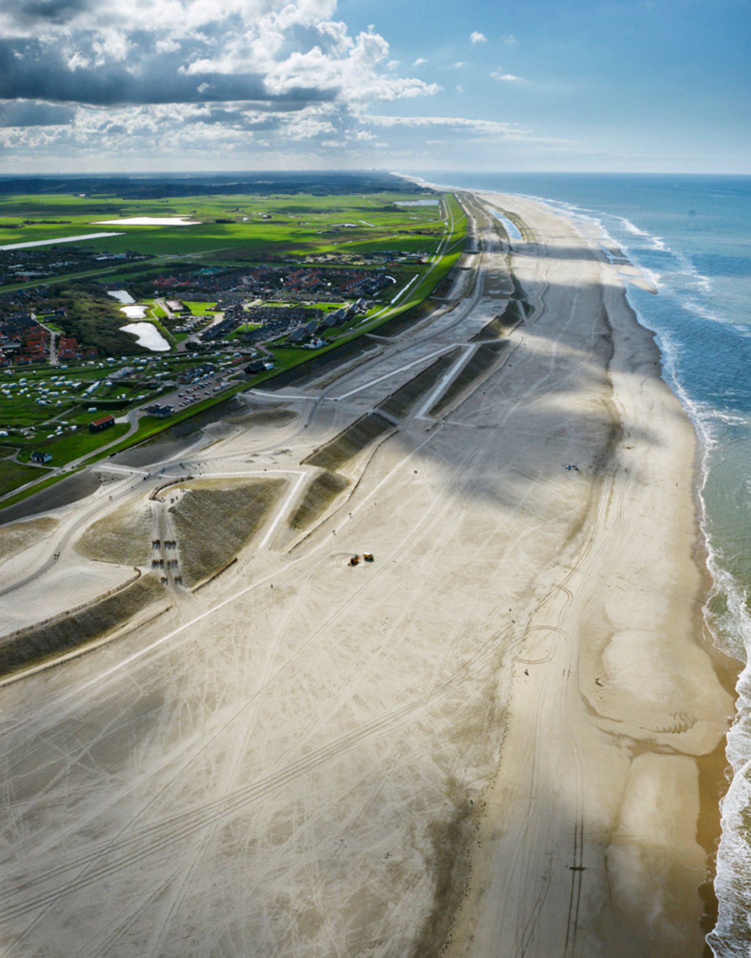
Hondsbossche Zeewering, Petten, North Holland: reinforcement of the sea dike, with dunes as natural flood defence measure and a beach for recreation. [© Aerophoto Schiphol]
