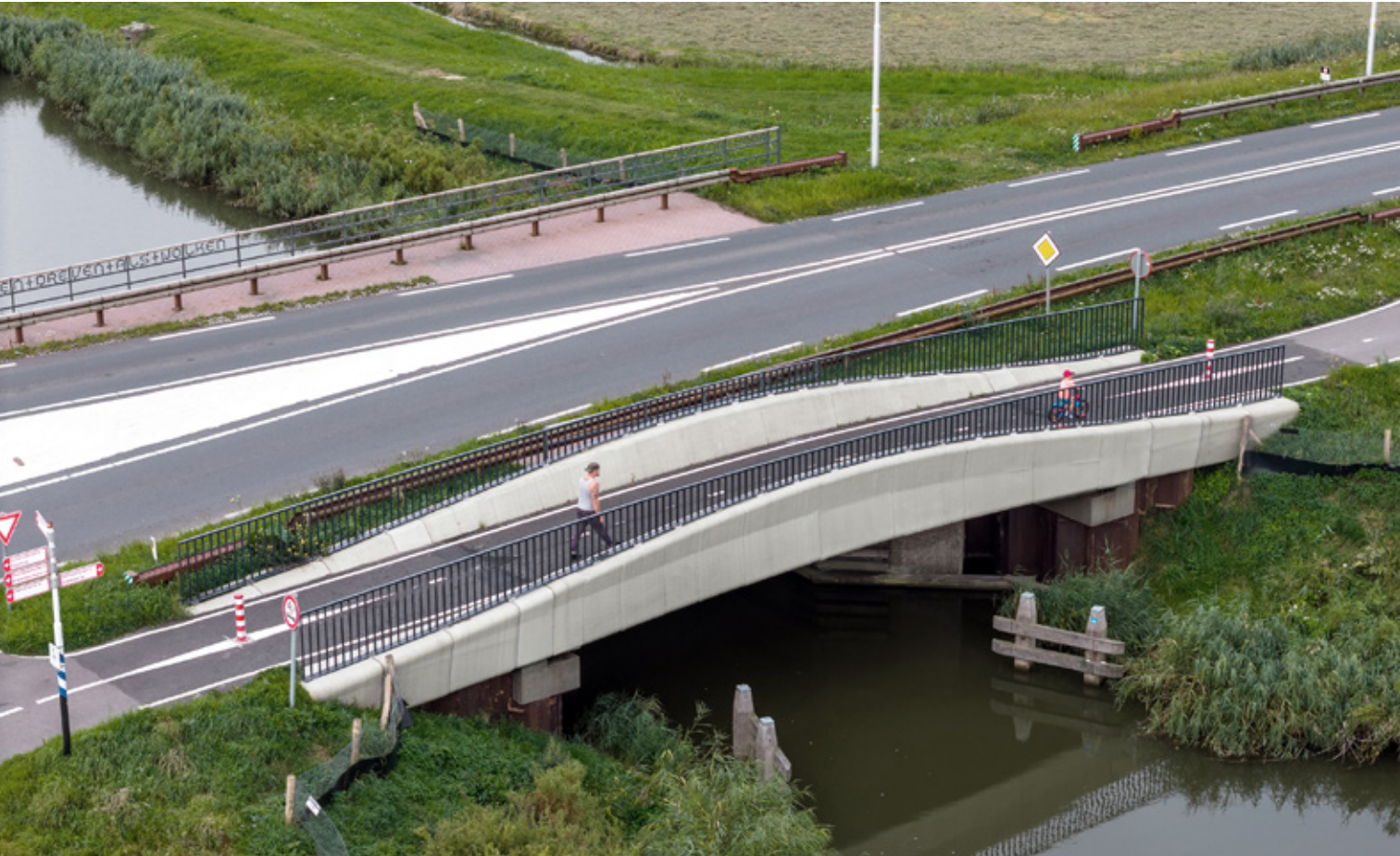
Deventer, Overijssel: new secondary canal in the floodplains of the IJssel River for extra discharge capacity combined with a marina. / North Holland: 3D printed concrete bicycle bridge for the reconstructed N243 road Alkmaar – Avenhorn. [© Witteveen+Bos]
