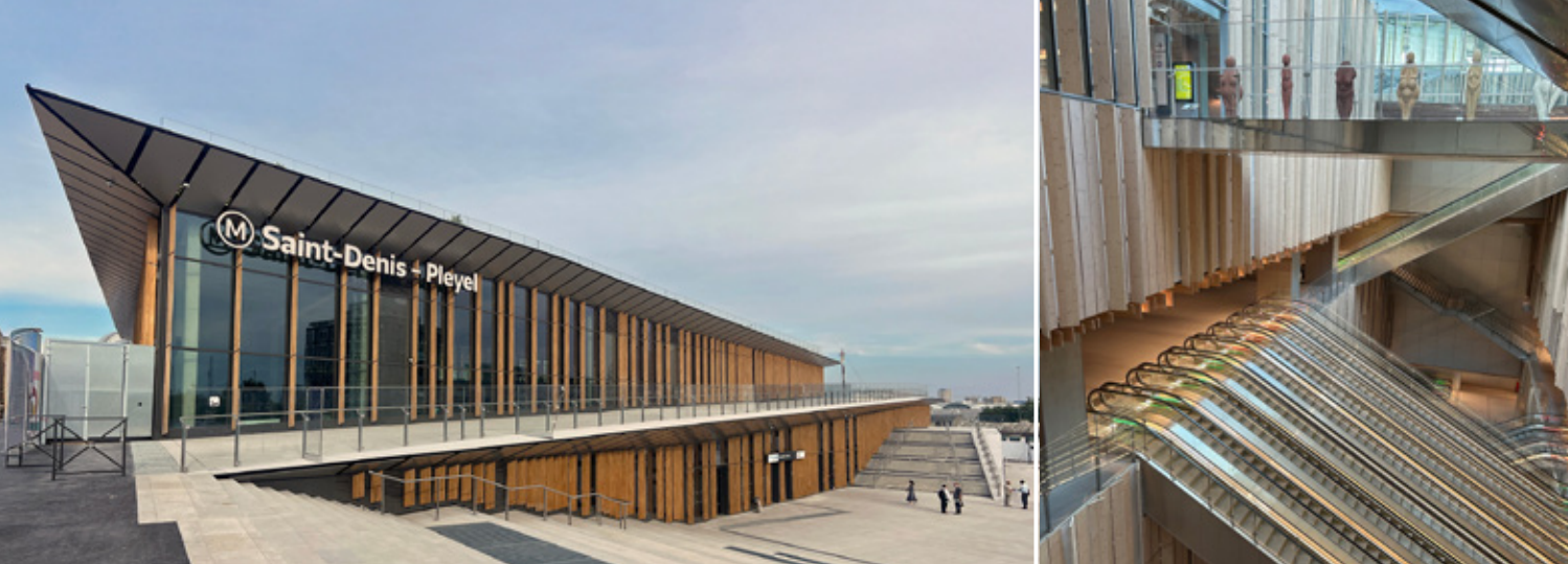
Figure 4. Grand Paris Express: metro station Saint-Denis – Pleyel, hub station for the lines 14, 15, 16 and 17. [CC Chabe01 / CC Chris93]
