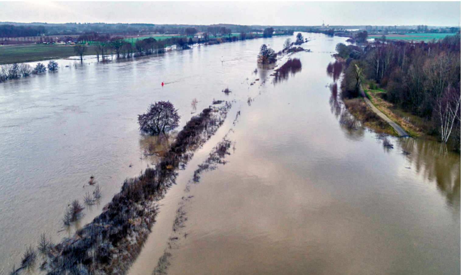
Figures 2–3. Well-Aijen Zuid, Limburg: high water discharge canal shown with the regular water level. [© Rijkswaterstaat, Joop van Houdt] / Discharge of high water via the discharge canal, February 2020. [© Rijkswaterstaat, Studio Retouched]
