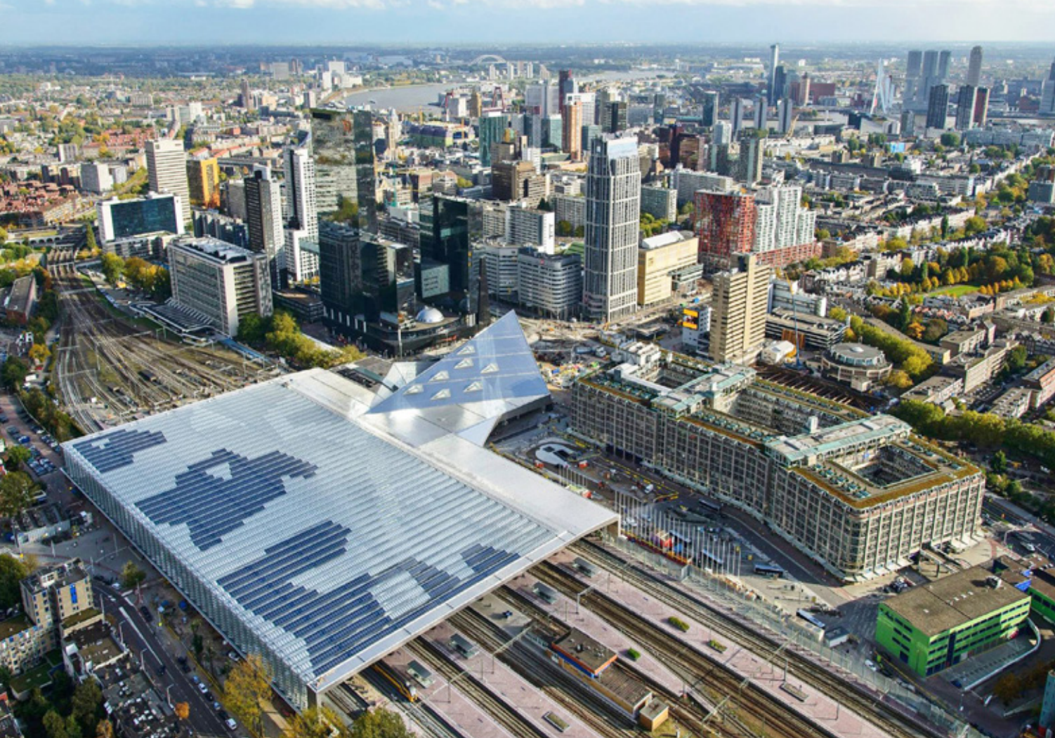
Figure 2. Rotterdam Centraal station within a high-density, mixed urban area as one of the six Dutch key projects for station renewal. [© Jannes Linders]
