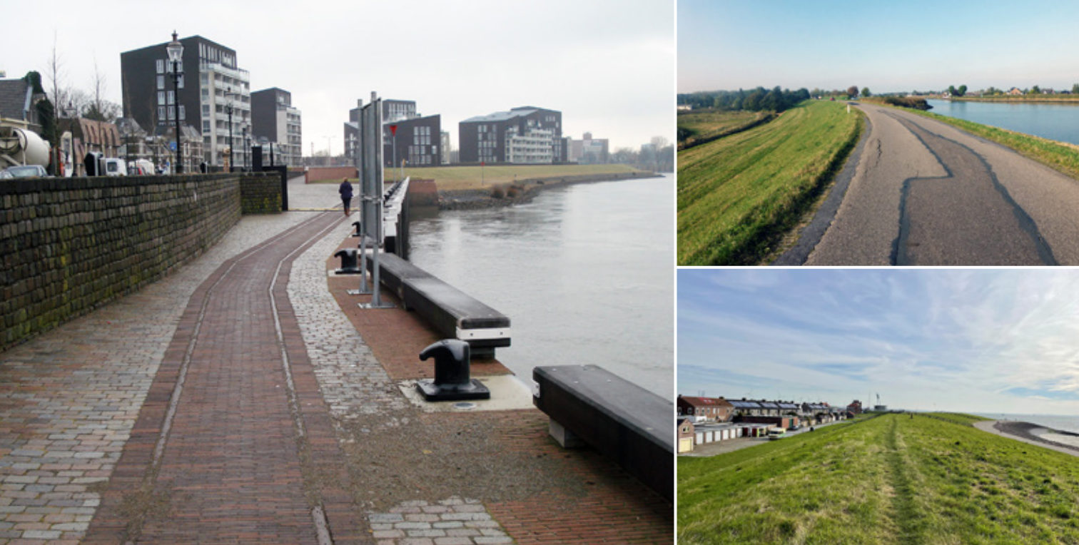
Doesburg, Gelderland: integration of flood defences in an urban context. [Mark Voorendt] / Top right: river dike along the Hollandse IJssel. [Mark Voorendt] / Vlissingen, Zeeland: sea dike. [Cong Mai Van] / Below: Deventer, Overijssel: multifunctional flood defence along the IJssel river. [Mark Voorendt]
