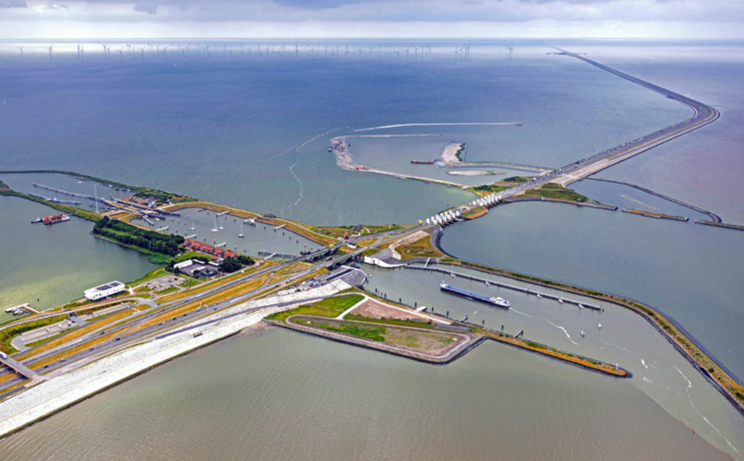
Reinforcement and renewal of the Afsluitdijk: Kornwerderzand sluice complex with sea lock, Lorentz sluice gates and the new Fish Migration River (under construction) as seen from the Wadden Sea. / Den Oever sluice complex with sea lock, two new pump stations, and additional sluice gates (under construction) next to the existing Stevin sluice gates, as seen from the IJsselmeer. [© Levvel, Topview Luchtfotografie]
