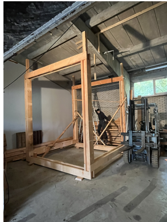
Prototyping the modular timber structure
