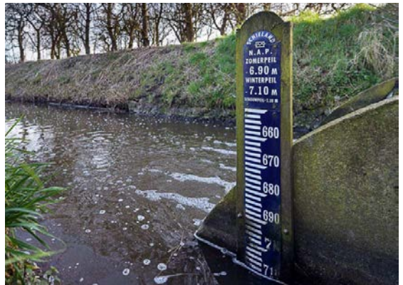
Water elements in the area
