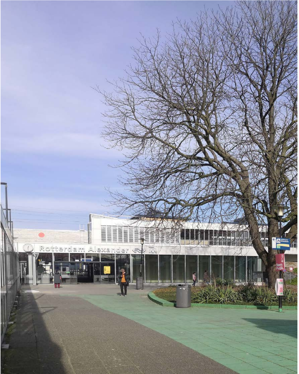
Rotterdam Alexander Station, Feb 2021
