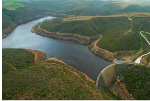
Figure 6.1. Wolwedans Dam, just upstream of Groot Brak Estuary (Source: DWS, South Africa)
