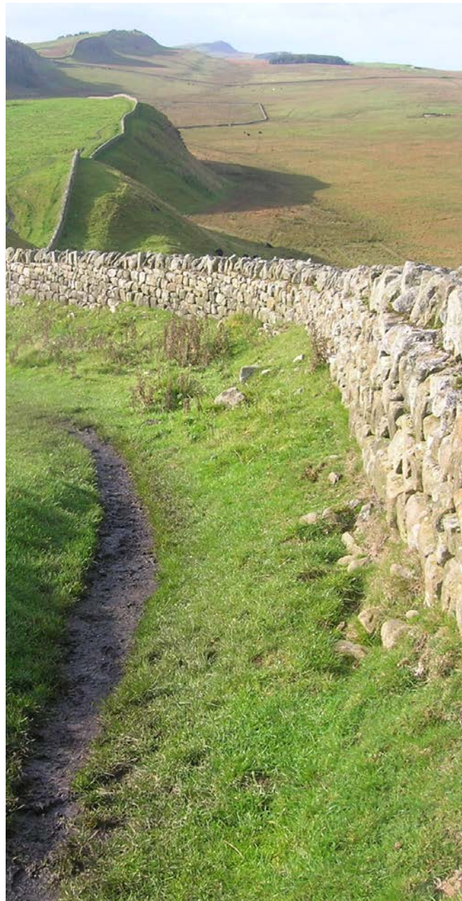
A VIEW OF HADRIAN'S WALL SHOWING ITS LENGTH AND HEIGHT. THE UPRIGHT STONES ON TOP OF IT ARE MODERN, TO DETER PEOPLE FROM WALKING ON IT. PHOTO BY QUISNOVUS, FROM GLOUCESTER, ENGLAND, CC BY 2.0. SOURCE: HTTPS://COMMONS.WIKIMEDIA.ORG/W/INDEX.PHP?CURID=101730445
