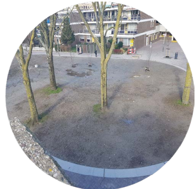
2. Green spaces are empty and poorly maintained
