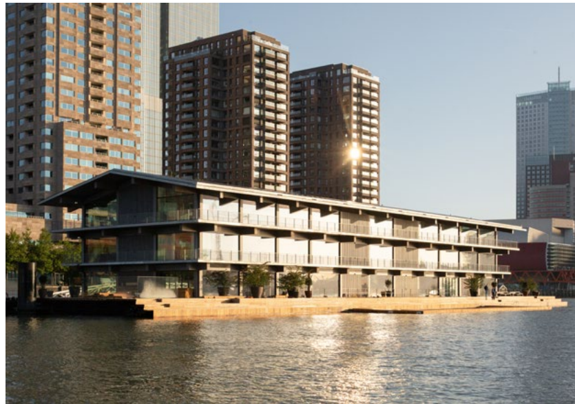
Figure 4 Where possible building on water utilizes otherwise neglected surface area and is future-proof, even with rising sea levels. The floating office featuring amongst others the Global Centre on Adaptation (design: Powerhouse Company) in the harbour of Rotterdam is the largest floating office in the world (3,600 m 2 ) (photograph by Marcel IJzerman).
