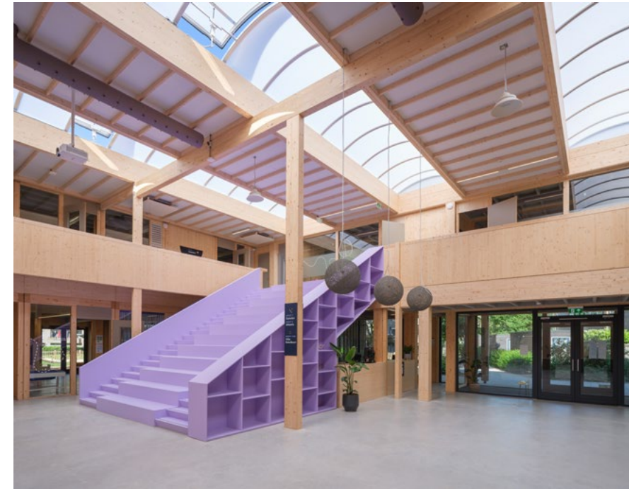
Figure 5 WThis school in Rotterdam (design: SeArch) was built within a very low budget and designed for disassembly with timber modules. It is planned to be rebuilt in five years in another location (photograph by Ossip van Duivenbode for SeArch).
