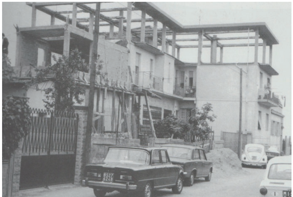
Fig. 3. The extension of a corea -house, a permanent non-finito state, 1973. Courtesy of Piero Airaghi.
