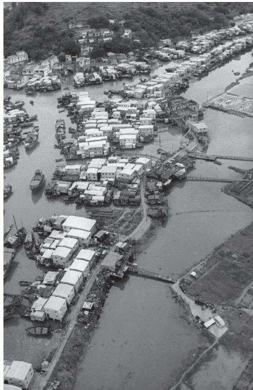
Figure 3. Tai O Village as seen in the 1972 aerial census, showing the stilt house districts and nearby shop houses. Source: Hong Kong Government Information Resources Department. Used with permission.
