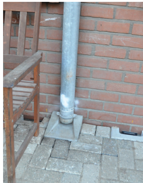
Disconnected drainpipes
