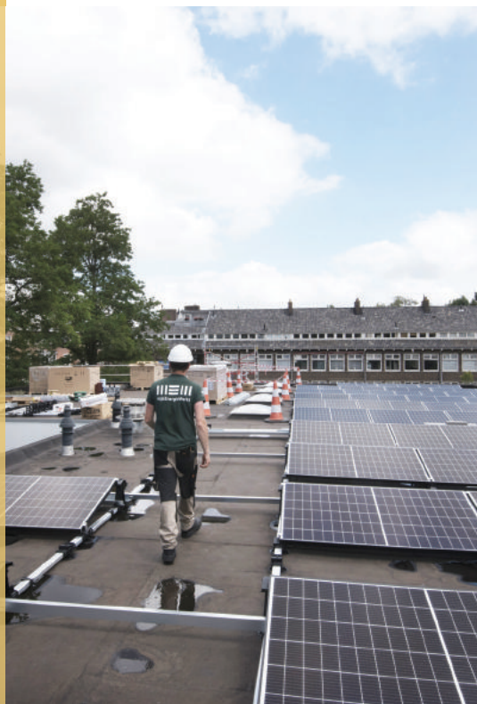
WijkEnergieWerkt employee on the solar roof being installed on Dalton school De Margriet
