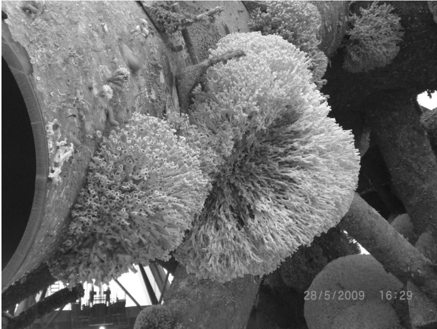
Fig. 5 Lophelia pertusa corals on the legs of the decommissioned platform North- West Hutton, North Sea. (BP)
