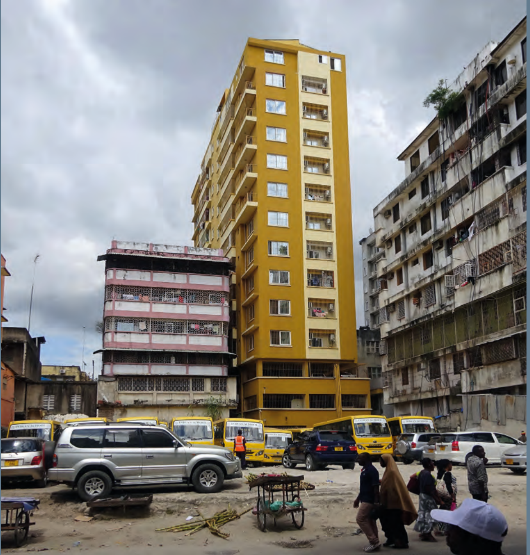
Central Dar es Salaam under redevelopment
