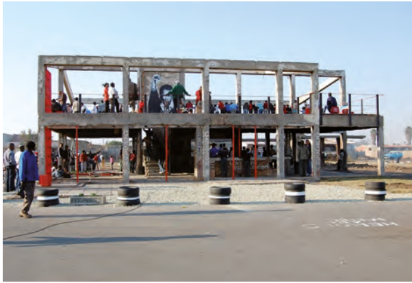
The KwaThema Project, beer hall reuse photo credit: Le Roux
